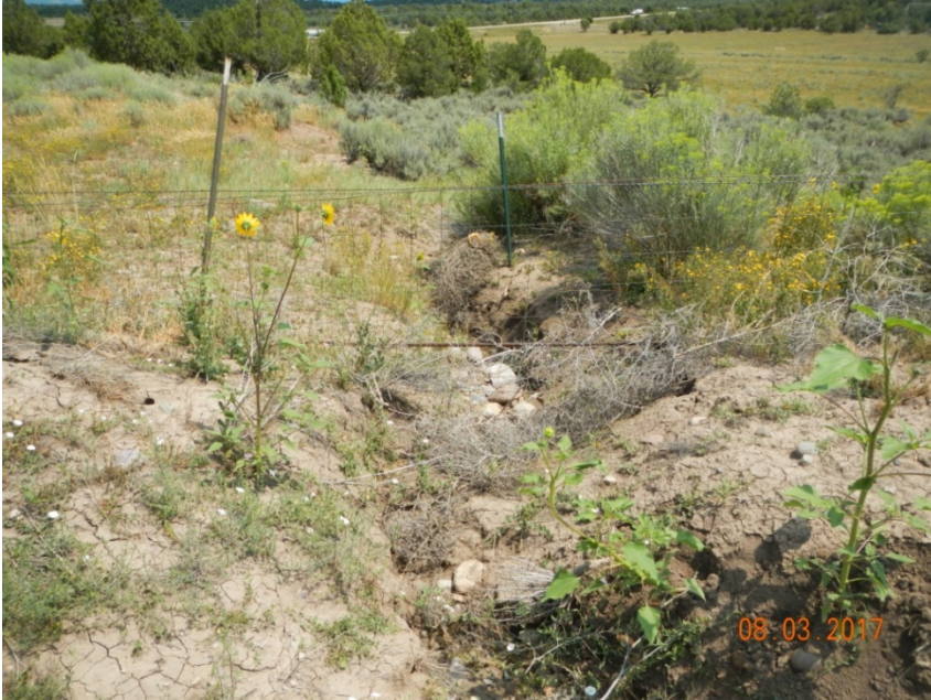
Photo 7: View of erosional channel in the northern portion of the project area needing stabilization measures.
