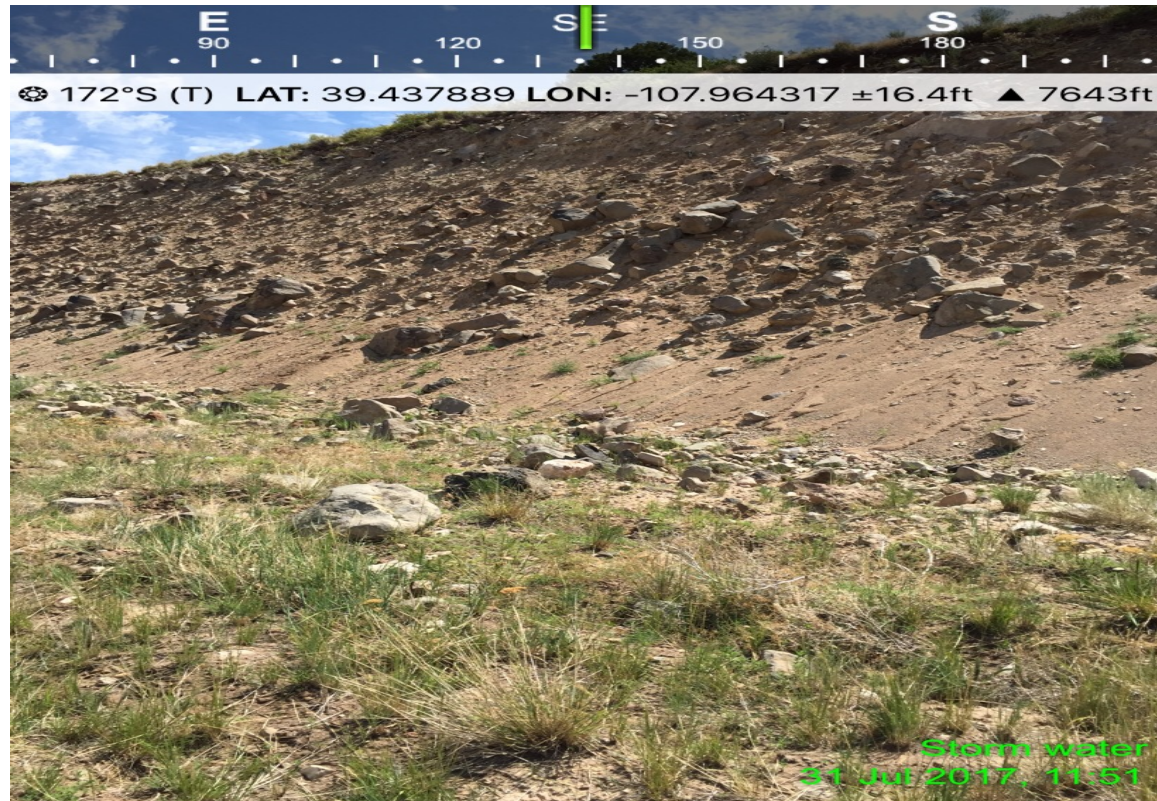
Photo 5. Cut slope not stabilized, debris and sediment moving onto pad
