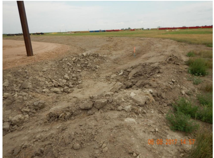
Photo 4. Photo taken from the southeast location, facing Northeast. Appears to be a sediment trap but no stabilized outfall protection has been installed. Embankment berms do not appear to be properly compacted.
