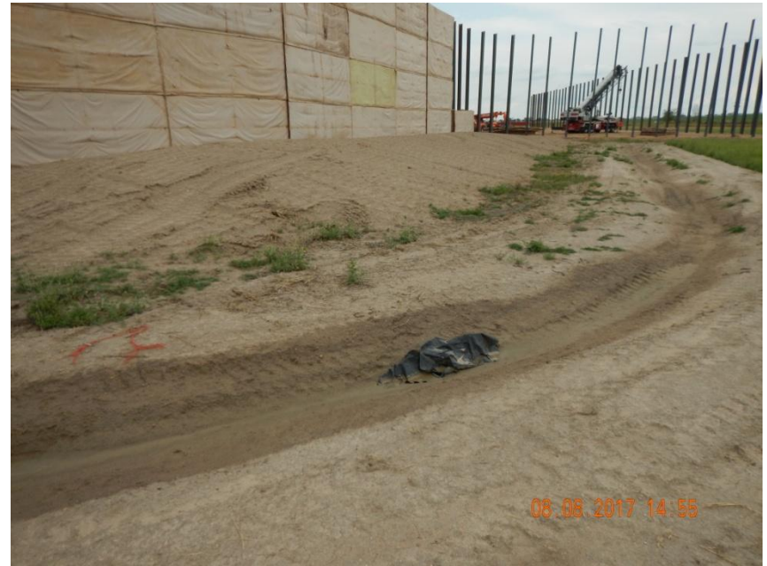
Photo 2. Photo taken from the southwest location, facing East. Topsoil stockpile temporarily stabilized with equipment tracking.
