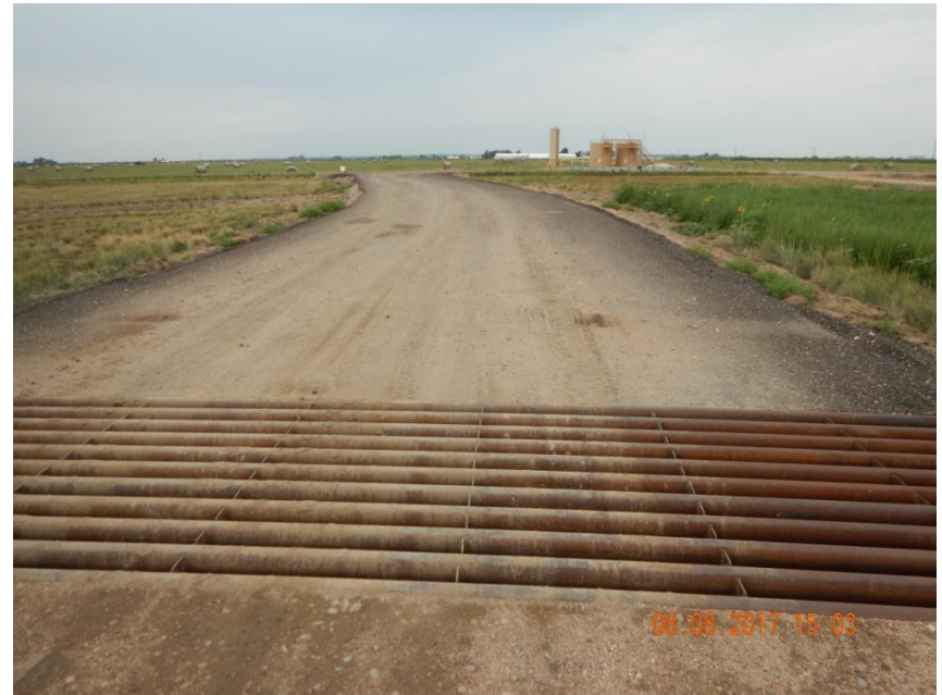
Photo 8. Photo taken from the entrance of the location, facing West. Vehicle tracking pad installed with a cattle guard.
