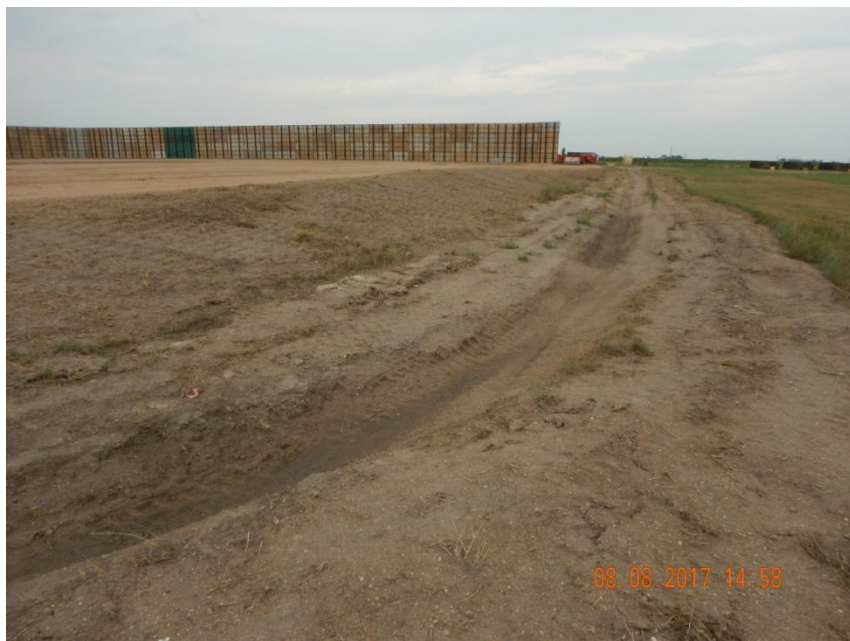
Photo 5. Photo taken from the southeast location, facing North. Ditch and berm BMP installed around the perimeter of the location. A second topsoil stockpile has been stored and temporarily stabilized with equipment tracking.
