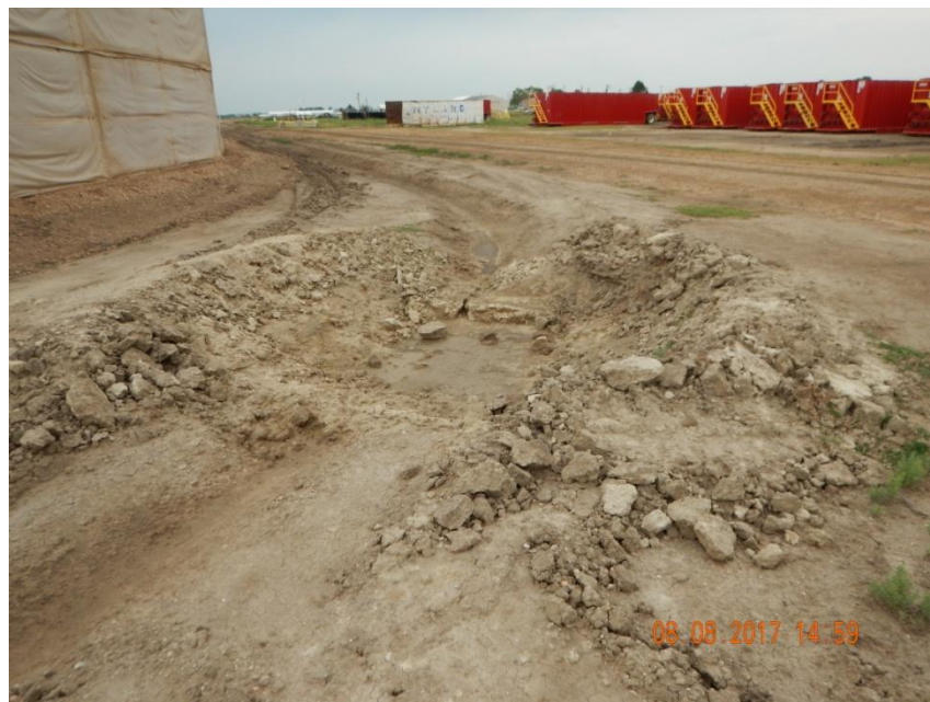
Photo 6. Photo taken from the northeast location, facing Northwest. Appears to be a sediment trap but no stabilized outfall protection has been installed. Embankment berms do not appear to be properly compacted.
