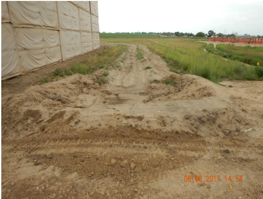
Photo 1. Photo taken from the western location, facing South. Appears to be a sediment trap but no stabilized outfall protection has been installed. Embankment berms do not appear to be properly compacted. Ditch and berm BMP installed around the perimeter of the location.
