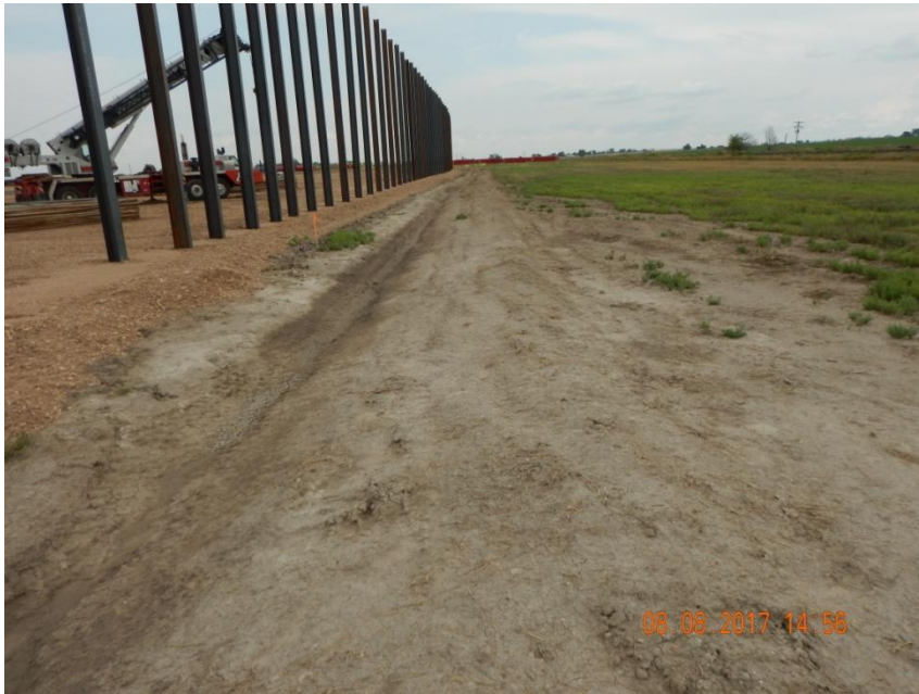
Photo 3. Photo taken from the southern location, facing East. Ditch and berm BMP installed around the perimeter of the location.
