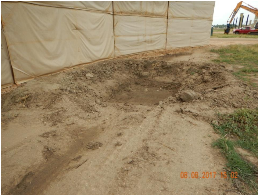
Photo 7. Photo taken from the western location, facing South. Appears to be a sediment trap but no stabilized outfall protection has been installed. Embankment berms do not appear to be properly compacted.
