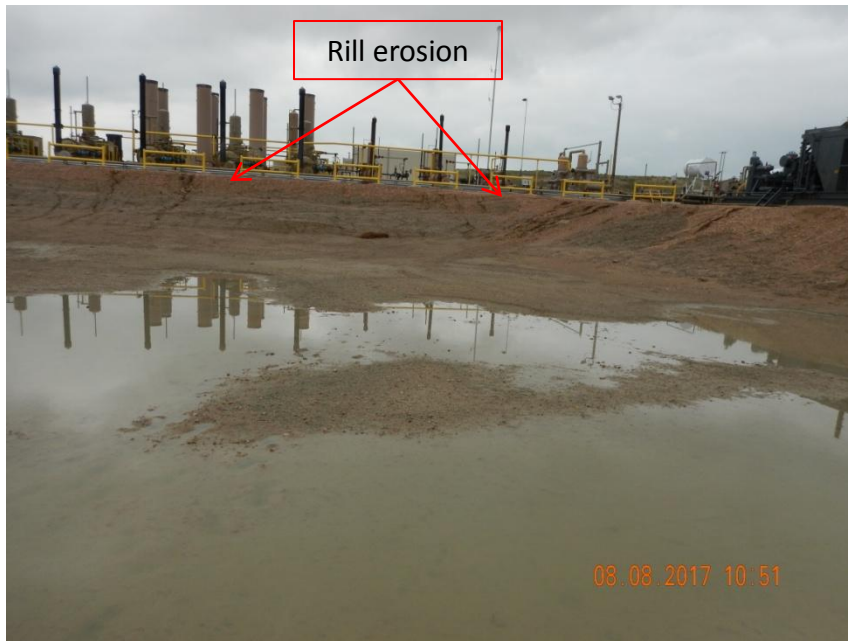
Photo 12. Photo taken from the Rancho Pad, facing South. Photo illustrates rill erosion occurring along the fill slopes of the production area.
