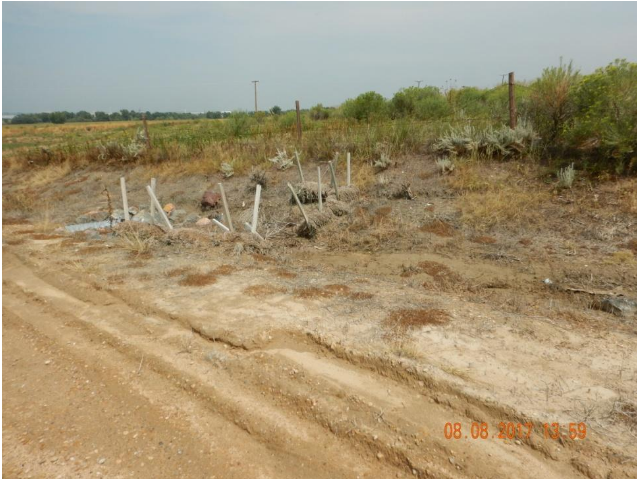
Photo 11. Photo taken from the eastern perimeter, facing Northeast. Stormwater BMPs for inlet protection are in need of maintenance.
