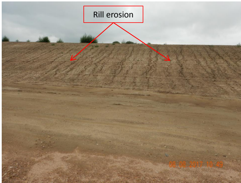
Photo 5. Photo taken from the northern location, facing South. This is the previously mentioned soil stockpile where rill erosion occurring and causing sedimentation at the toe of the soil stockpile. Soil stockpile needs to be stabilized to prevent rill erosion.
