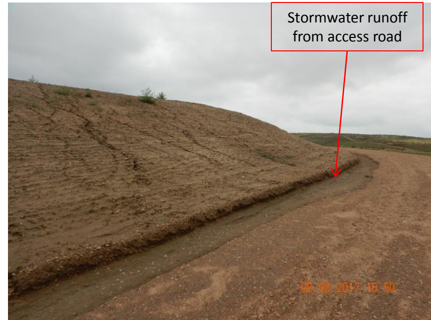
Photo 6. Photo taken from a portion of the access road, facing Southwest. This is the previously mentioned access road where stormwater runoff is traveling along the access road along the toe of the soil stockpile. Soil stockpile needs to be stabilized to prevent rill erosion.
