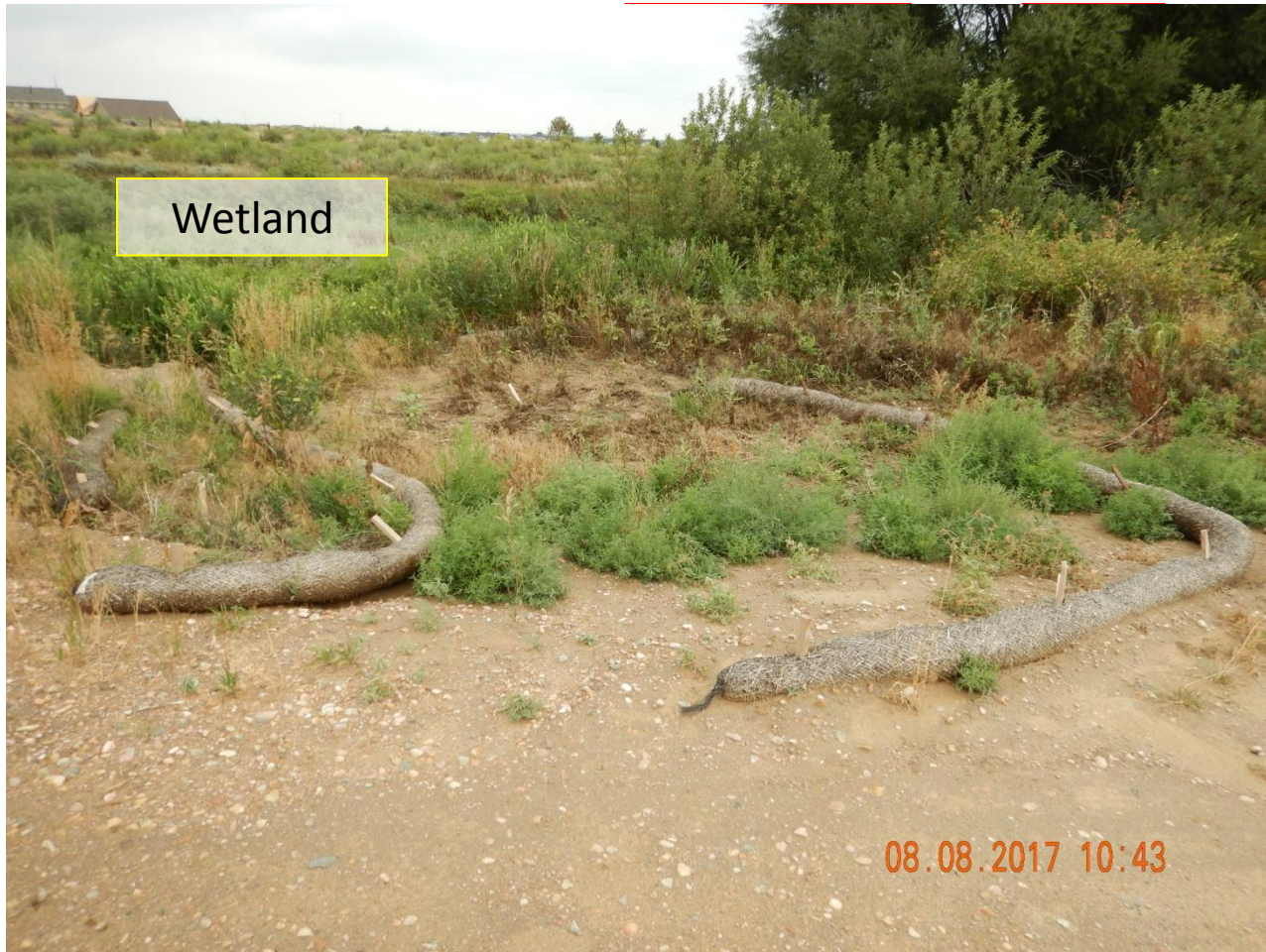
Photo 3. Photo taken from the area of erosion, facing North. Photo illustrates stormwater runoff that has caused wattle BMPs to dislodge and cause gully erosion. Operator claims these wattle BMPs are not theirs because it is off location and that the wattle BMPs are DCPs.
