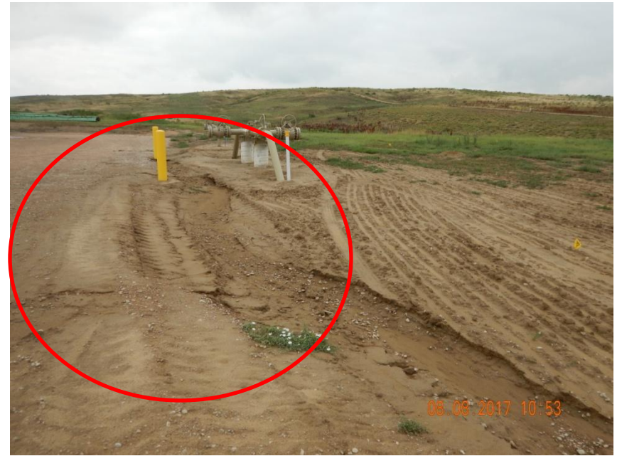
Photo 10. Photo taken from the western Rancho Pad, facing South. Photo illustrates stormwater erosion coming from the Rancho Pad and causing erosion off location.
