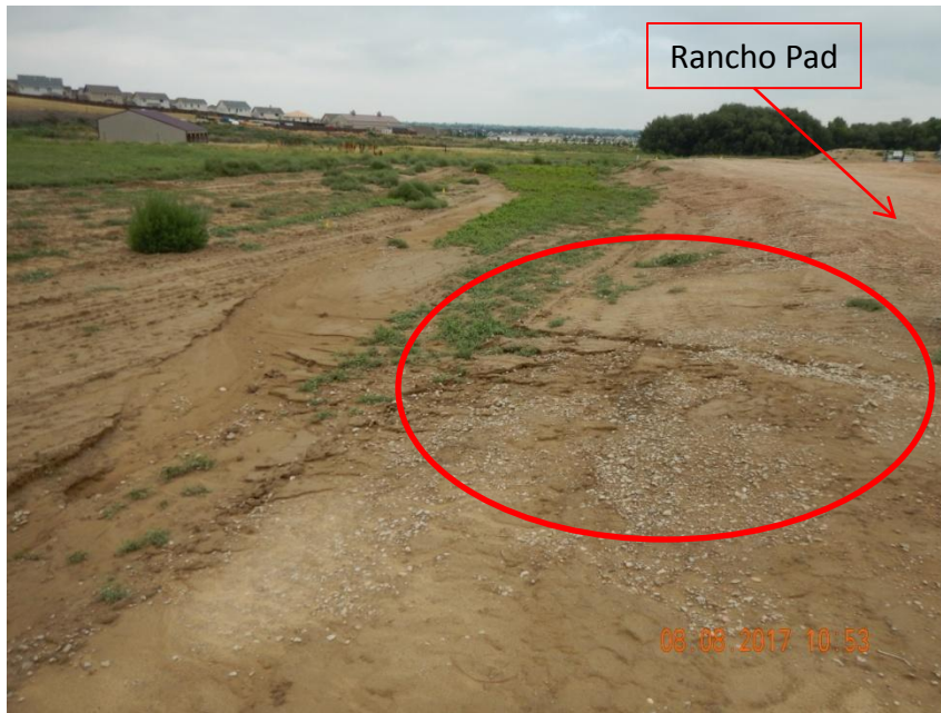
Photo 9. Photo taken from the western Rancho Pad, facing North. Photo illustrates stormwater erosion coming from the Rancho Pad and causing erosion off location.
