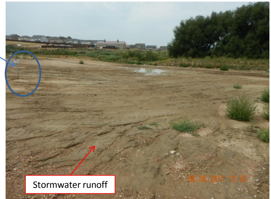
Photo 8. Photo taken from an eastern portion of a DCP pipeline area, facing West. Photo illustrates stormwater runoff coming from the access road of the Rancho Pad off location.
