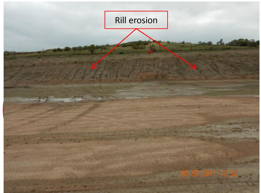
Photo 13. Photo taken from the eastern Rancho Pad, facing East. Photo illustrates rill erosion occurring along the cut slopes.
