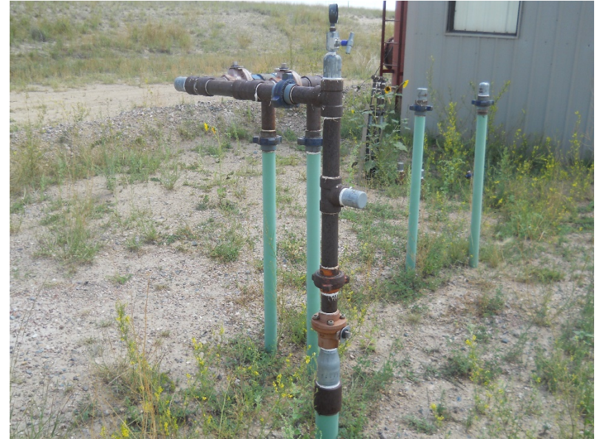
3-2" Risers plumbed in to each other north side of heater treater
