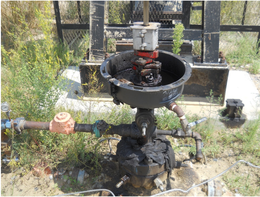
Pump jack looking east, open top container containing fluid with no wildlife protection. Stained soil around wellhead
