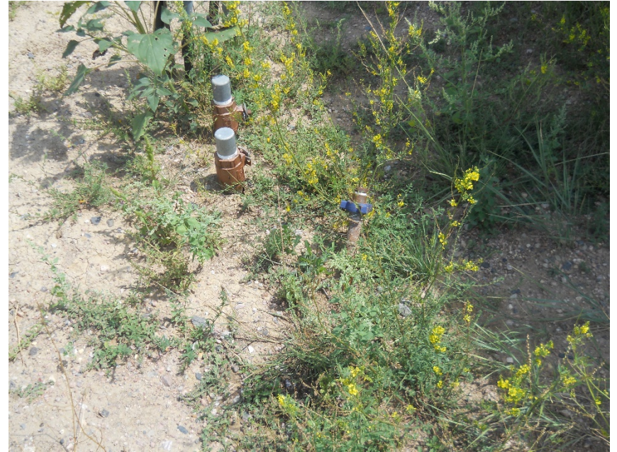
1-1" unused/unmarked riser north side of heater treater shed 2-2" unused/unmarked risers north side of heater treater shed
