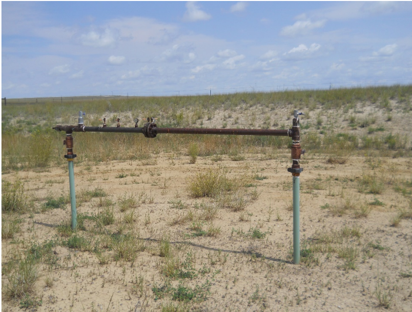
Unused meter run set with no meter
