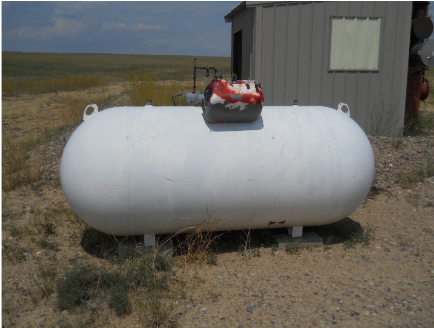
Propane tank with no labeling , south side
