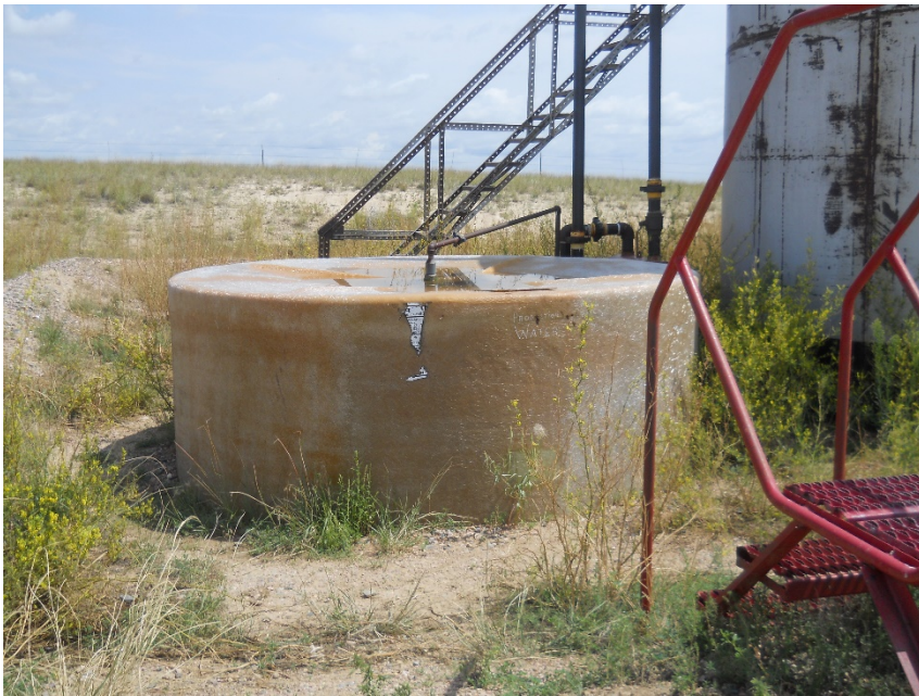
Water tank missing capacity, NFPA label. Production water written on tank but hard to read.
