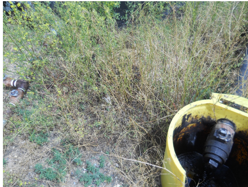
Stained soil around load line bucket on southwest tank. Top of load line bucket is not in place, standing fluid inside with no wildlife protection
