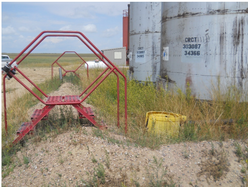
South side of tank battery looking north. Actively growing weeds inside and around tanks. Southwest tank does not have contents/capacity labeled
