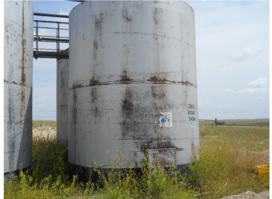
Southwest oil tank missing contents/capacity label
