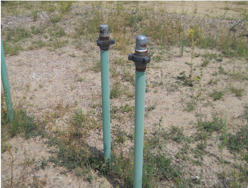
2-2" unused/unmarked risers north side of heater treater shed
