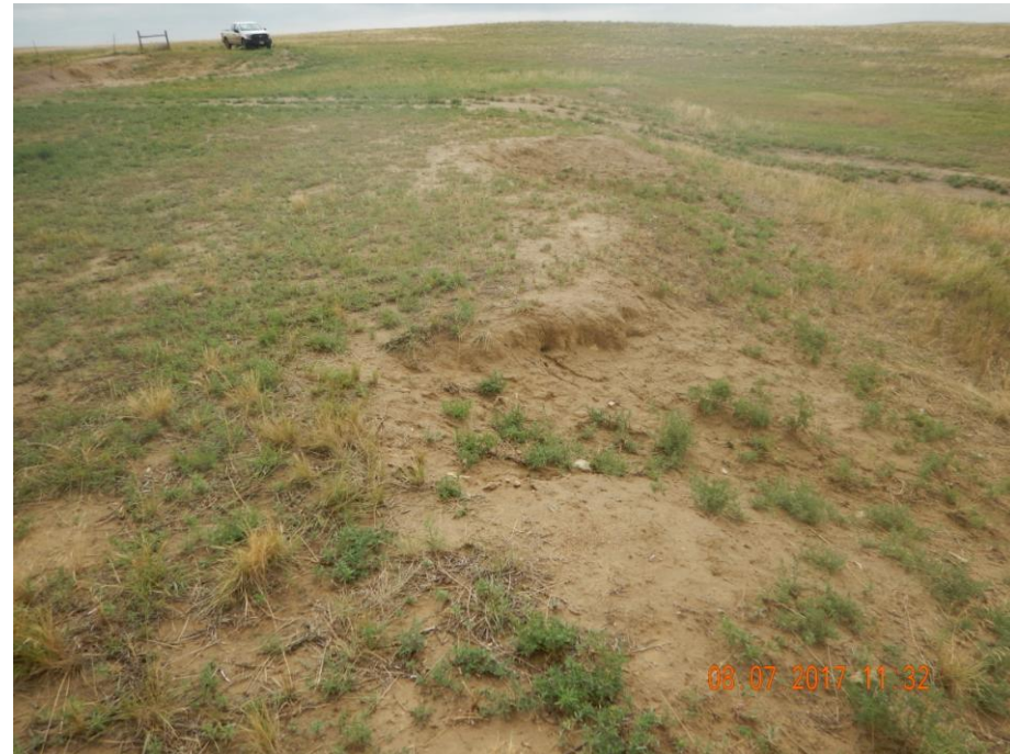
Photo 8: Photo taken from the south end of the location, facing east. Photo shows erosion degradation on the location has not been repaired, and stormwater and sediment control BMPs have not been installed.
