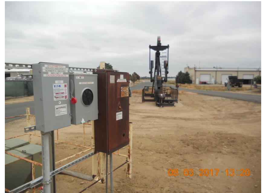
Photo 4. Electrical panels and transformers west of well. Note no meter installed
