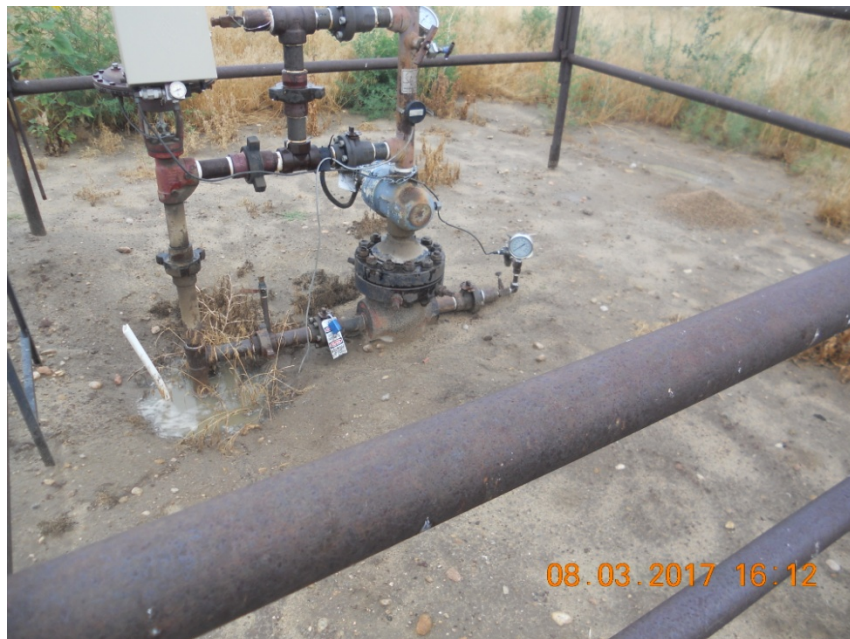
Photo 9. Wellhead looking east. Note casing valve LO/TO
