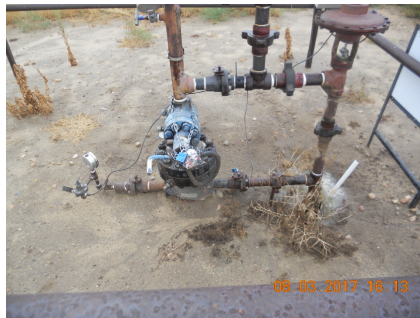
Photo 10. Wellhead looking west. Note master valve LO/TO
