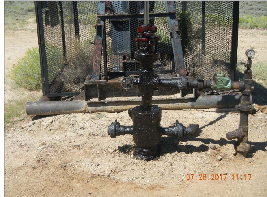
Photo 2. Leak at wellhead.
