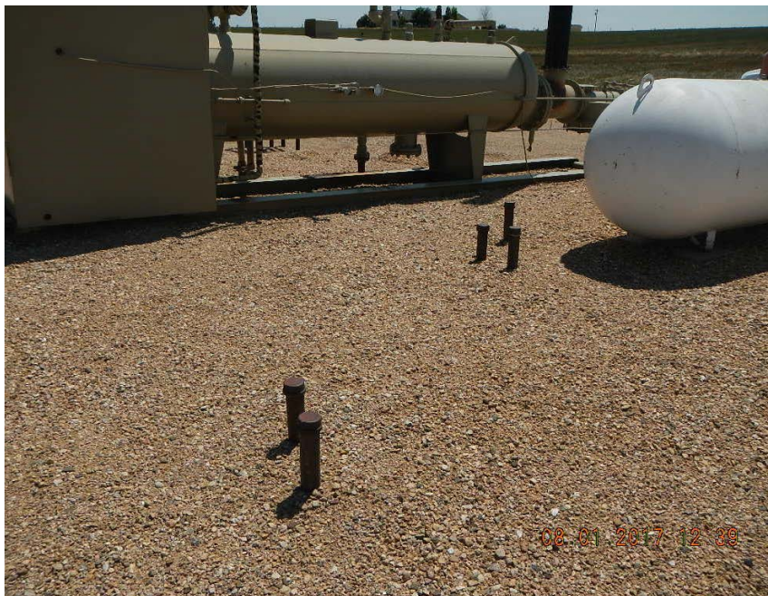
Unmarked 2" steel risers at separator
