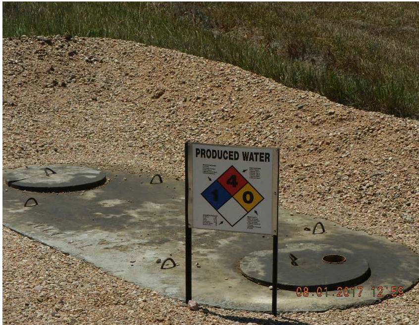
Produced water vault placarding
