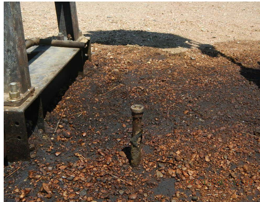
Unmarked 1" steel riser at wellhead
