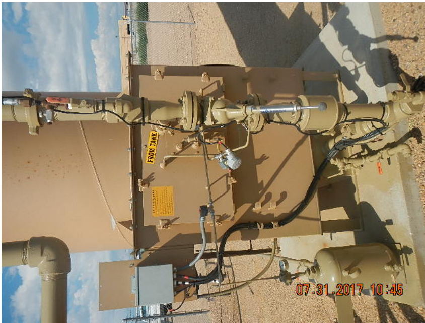
ECD BY PASSED FROM TANKS SHUT IN VALVE IN OPEN POSITION
