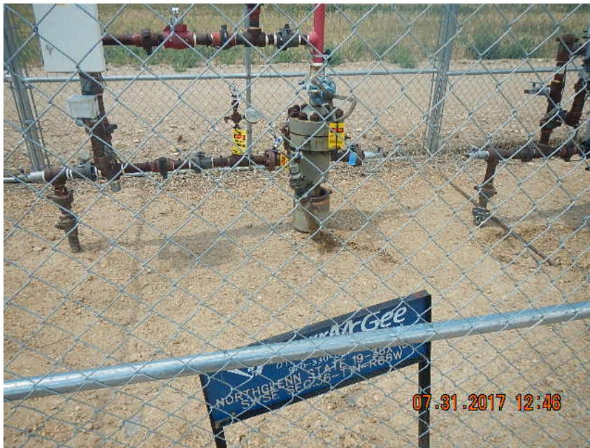
STAINED SOIL AT WELLHEAD
