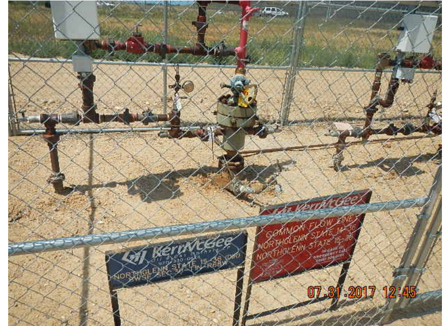
STAINED SOIL AT WELLHEAD
