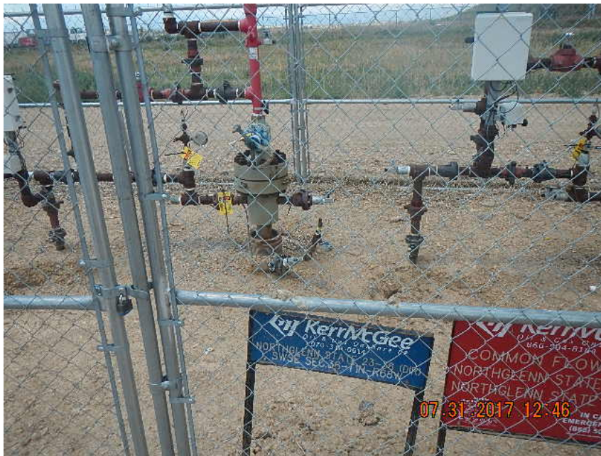
STAINED SOIL AT WELLHEAD
