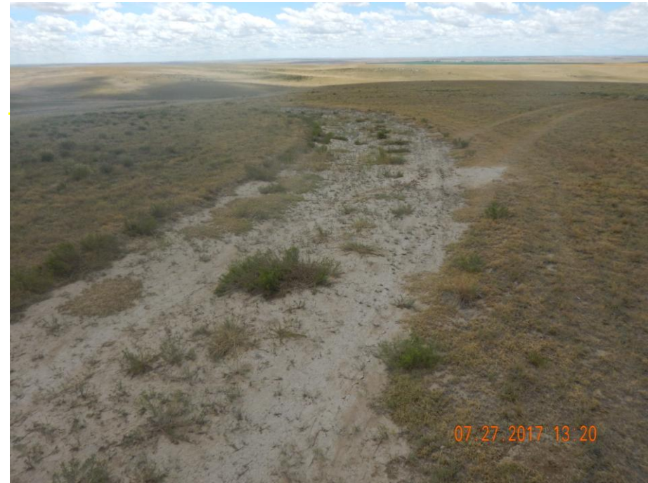
Photo 6: Photo taken from the access road on the northwest end of the well location. Photo shows access road still requires compaction alleviation, re-contouring, re-grading and re-vegetating
