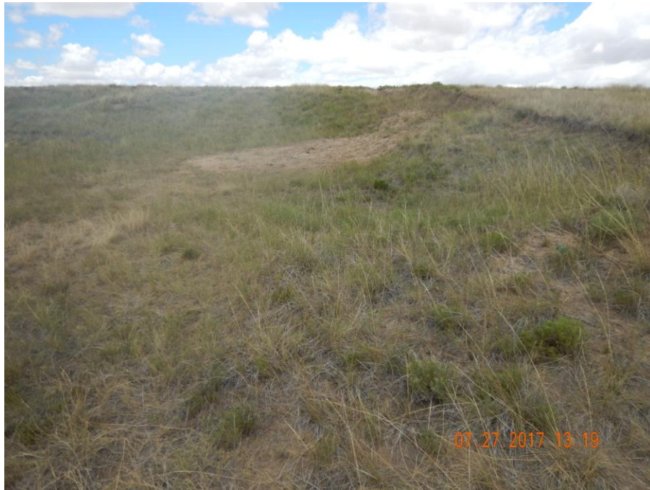
Photo 5: Photo taken from the northeast end of the well location, facing north. Photo shows location still appears to require re-contouring and re-grading.
