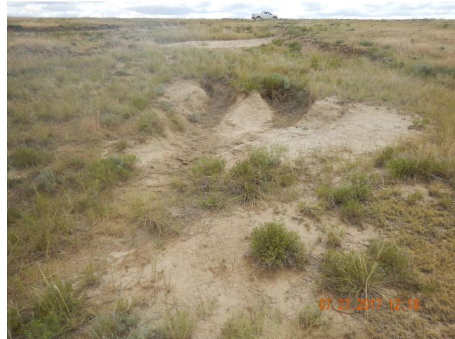
Photo 6: Photo taken from the down slope on the northern disturbance area, facing east towards the access road. Photo shows erosion has not been stabilized, not BMPs have been installed and/or maintained. No evidence of any additional remediation or reclamation efforts observed.
