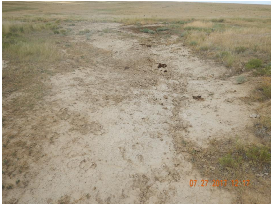
Photo 5: Photo taken from the down slope on the northern disturbance area, facing east towards the access road. Photo shows erosion has not been stabilized, not BMPs have been installed and/or maintained. No evidence of any additional remediation or reclamation efforts observed.
