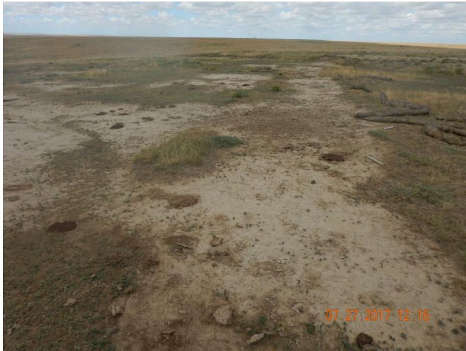
Photo 3: Photo taken from the northern disturbance area, facing north. Photo shows erosion has not been stabilized, not BMPs have been installed and/or maintained. No evidence of any additional remediation or reclamation efforts observed. Straw wattles observed in photo appear to be same wattles from previous inspections up to and over a year ago. BMPs in disrepair and is now debris.
