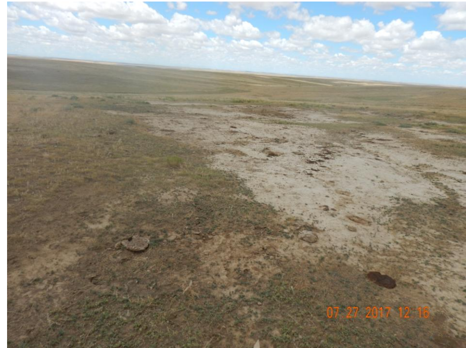
Photo 4: Photo taken from the northern disturbance area, facing west. Photo shows erosion has not been stabilized, not BMPs have been installed and/or maintained. No evidence of any additional remediation or reclamation efforts observed. Straw wattles observed in photo appear to be same wattles from previous inspections up to and over a year ago. BMPs in disrepair and is now debris.
