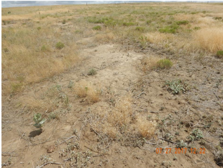
Photo 9: Photo taken from the down slope on the southern disturbance area, facing east towards the access road. Photo shows areas of the disturbance that remain un-vegetated and un-stabilized. No evidence of any additional remediation or reclamation efforts observed.
