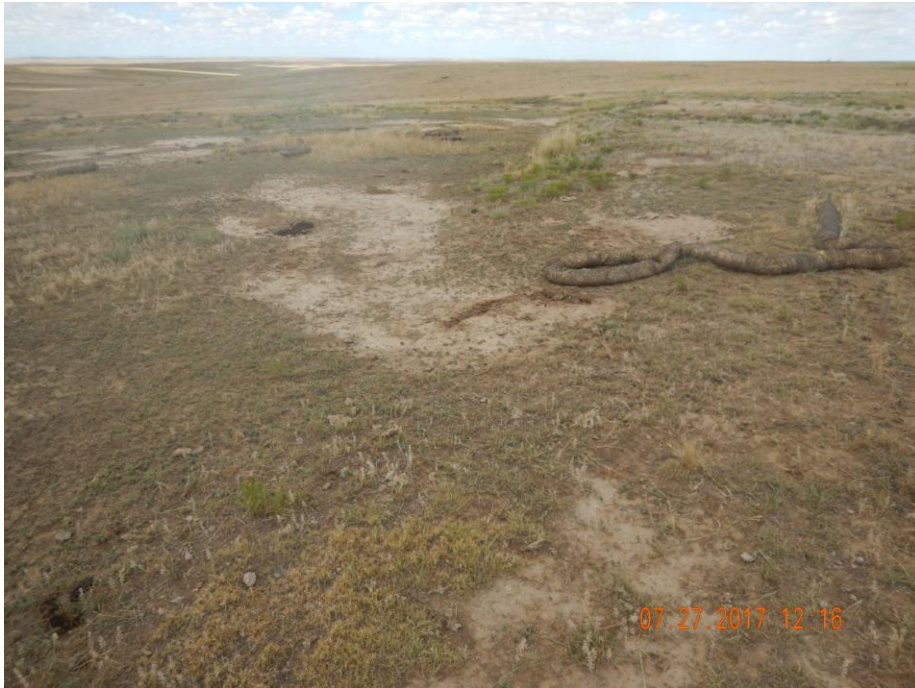
Photo 1: Photo taken from the northern disturbance area, facing northwest. Photo shows erosion has not been stabilized, not BMPs have been installed and/or maintained. No evidence of any additional remediation or reclamation efforts observed. Straw wattles observed in photo appear to be same wattles from previous inspections up to and over a year ago. BMPs in disrepair and is now debris.
