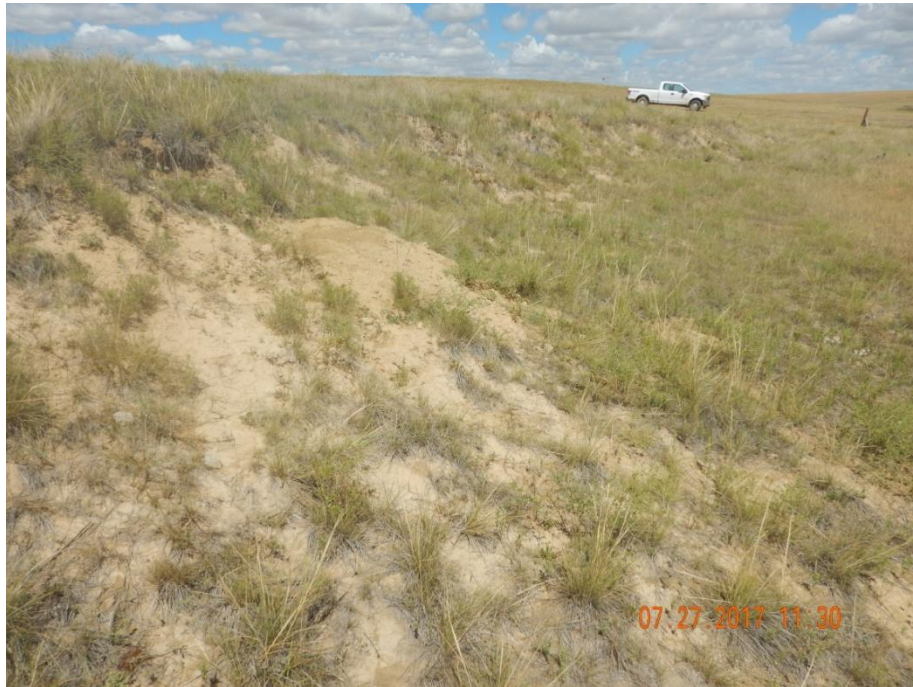
Photo 3: Photo taken from the southwest corner of the location, facing northwest. Photo shows erosion on cut bank. Photo shows location has not been re-contoured per CA's
