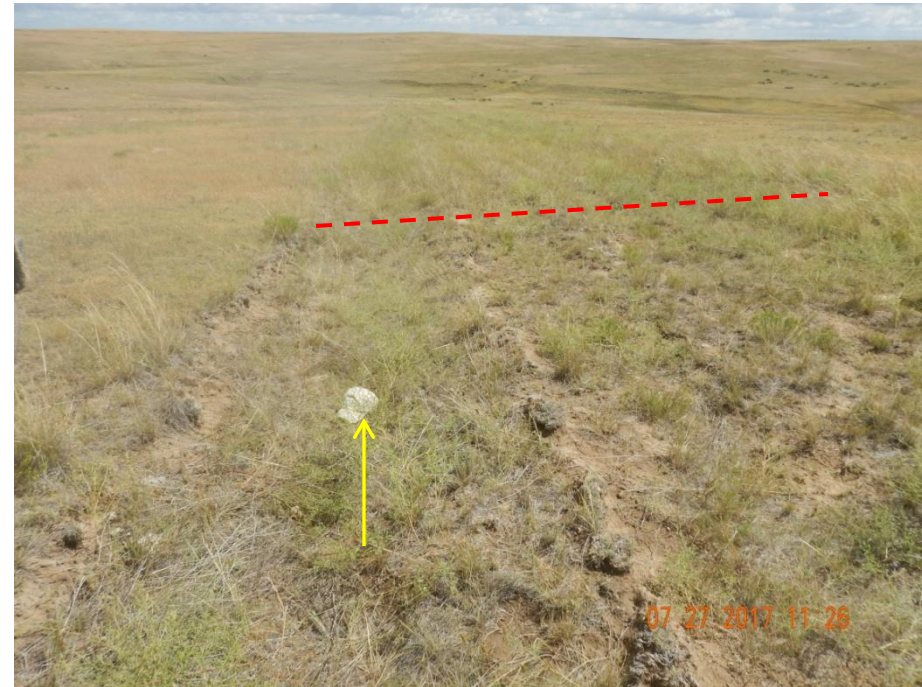
Photo 4: Photo taken from access road southeast of the location, facing north. Photo shows access road had not been re-contoured or re-graded as required per CA's. Hat (indicated by yellow arrow) used for reference. Red line indicates width of road.
