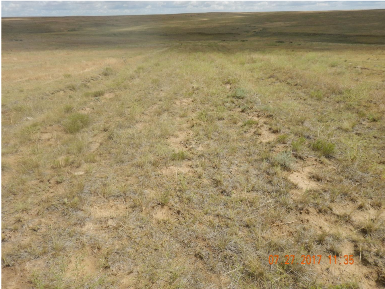
Photo 5: Photo taken from access road southeast of the location, facing north. Photo shows access road had not been re-contoured or re-graded as required per CA's.
