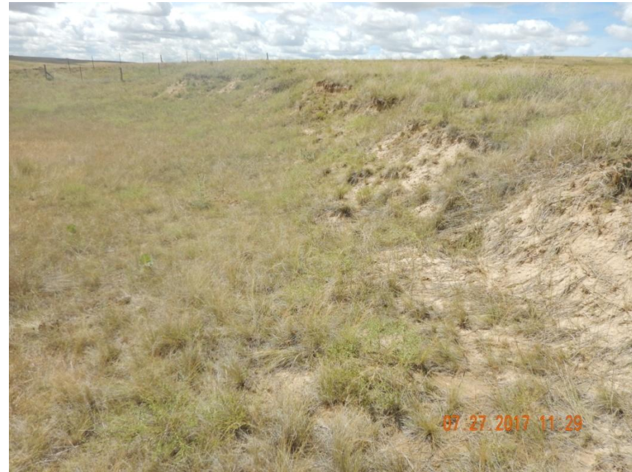
Photo 2: Photo taken from the west end of the location, facing southeast. Photo shows erosion on cut bank. Photo shows location has not been re-contoured per CA's
