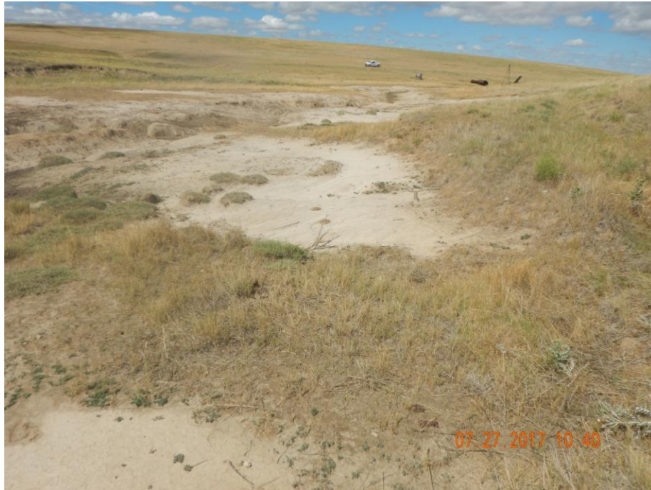
Photo 5: Photo taken from the north side of the drainage, adjacent to the pit and well location, facing west. Photo shows area of degradation that remain un-stabilized. Further degradation since previous inspection evident. See photos from inspection doc. # 682500927 for additional details.
