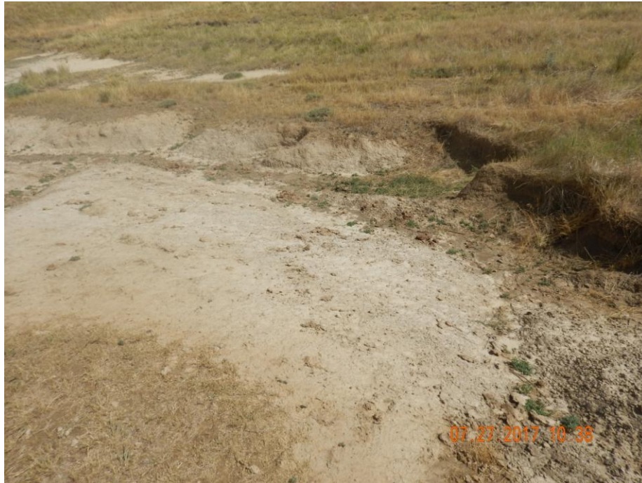
Photo 1: Photo taken from the south side of the drainage, adjacent to the pit and well location, facing north. Photo shows area of degradation that remain un-stabilized. Further degradation since previous inspection evident. See photos from inspection doc. # 682500927 for additional details.
