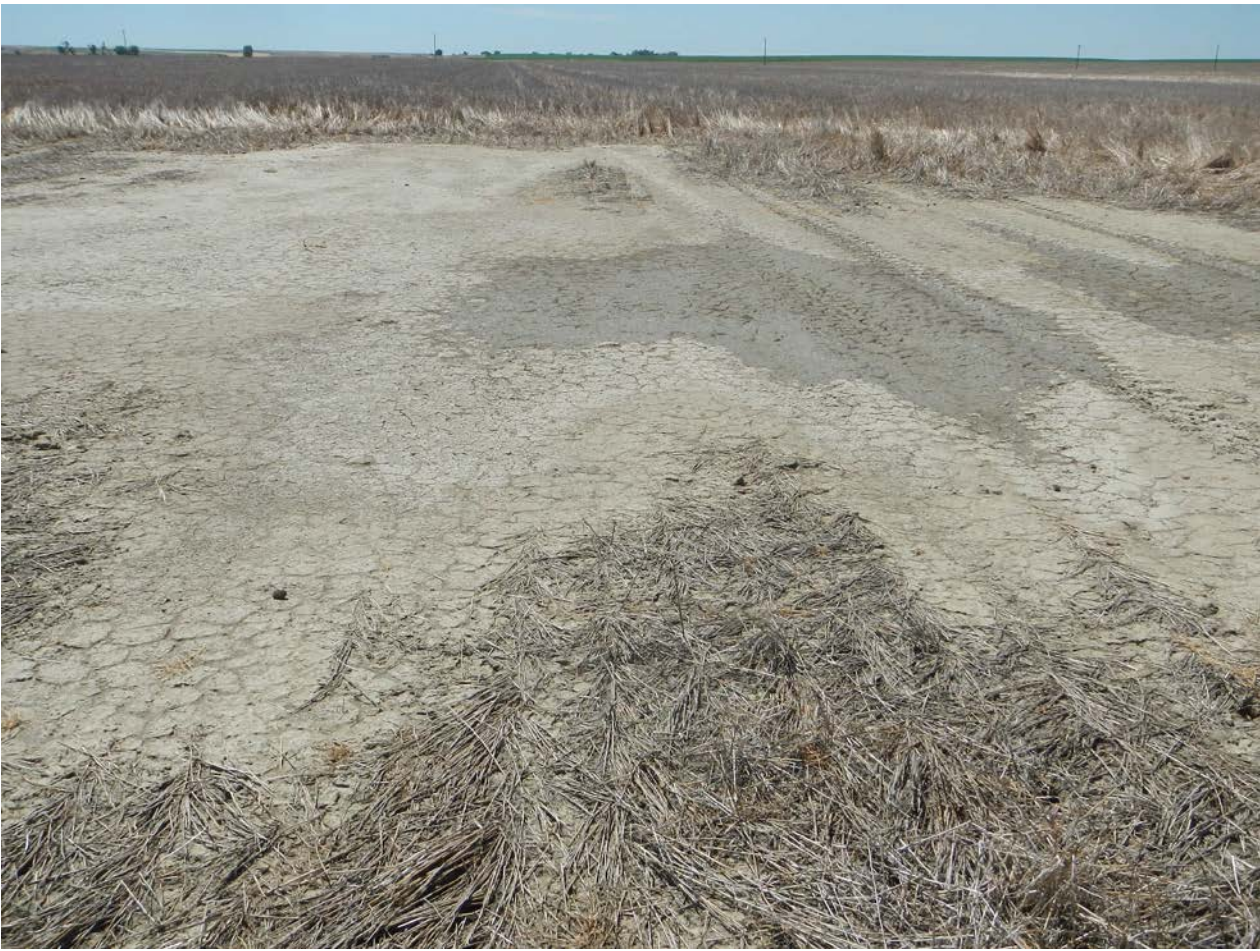
View south across pit, mud cracks and puddled water indicate subsidence and lack of crop growth.
