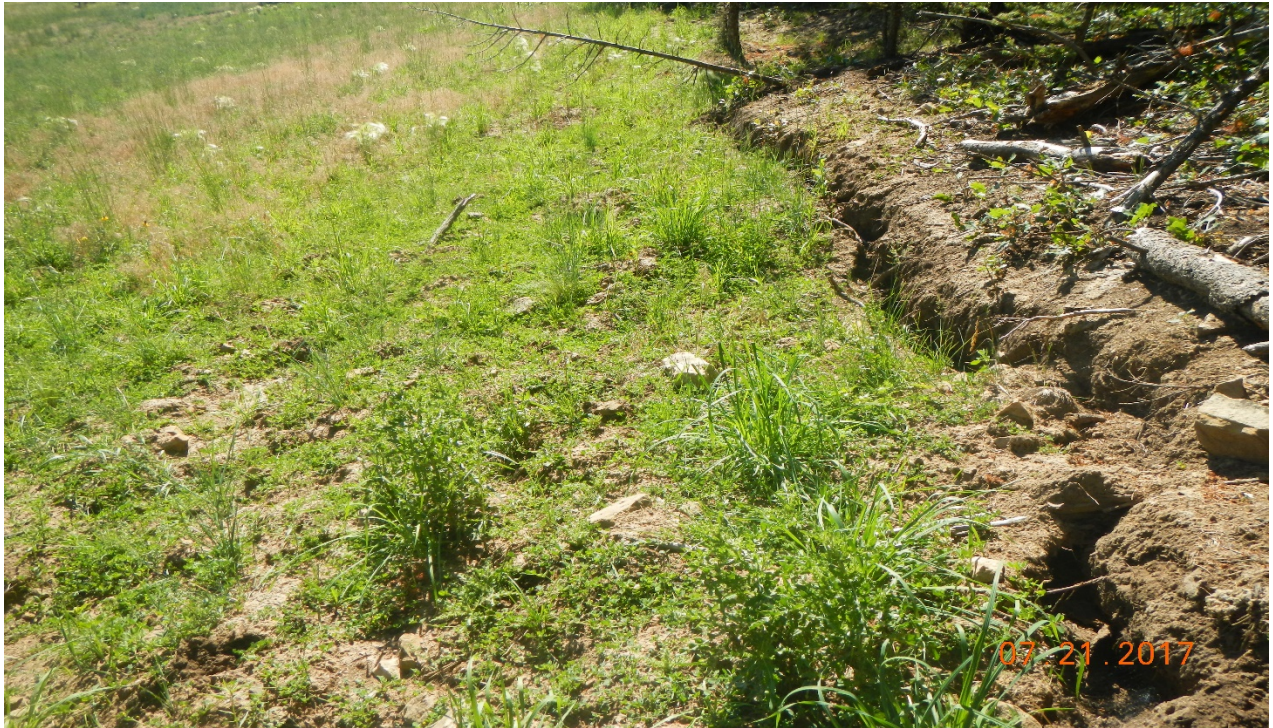
photo 9: There is subsidence occurring along the south side where soil was placed into the cut slope.
