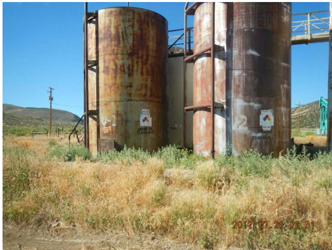
Tank battery with berm and vegetation (weeds).
