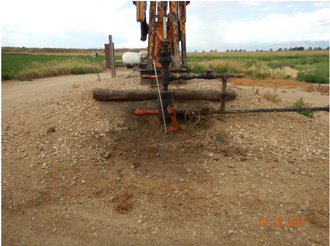
Figure 1 – Oil-stained soil, uncapped equipment, and flowline risers at wellhead. Note: Trailer, electrical boxes, and additional junk in background.
