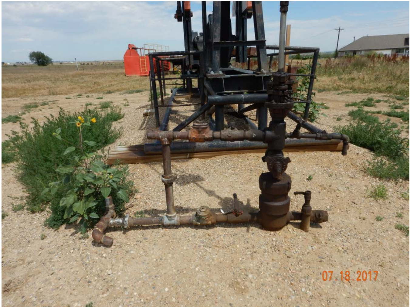
Photo 2 – Localized, oil stains on wellhead equipment, note COGCC tag with instructions not to operate remains attached.
