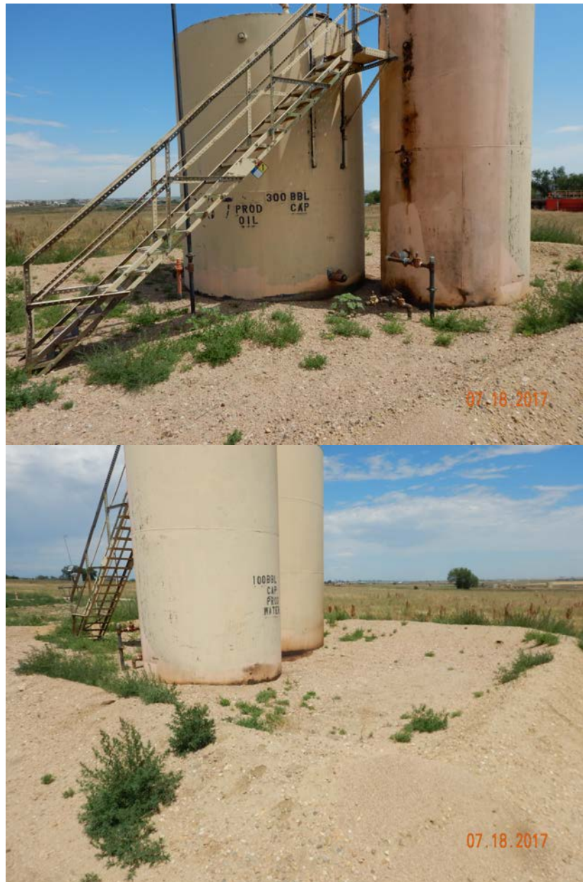
Photos 4 & 5- Tank battery with earthen berm, note fluorescent paint on abandoned flowline riser beside crude oil AST (top).
