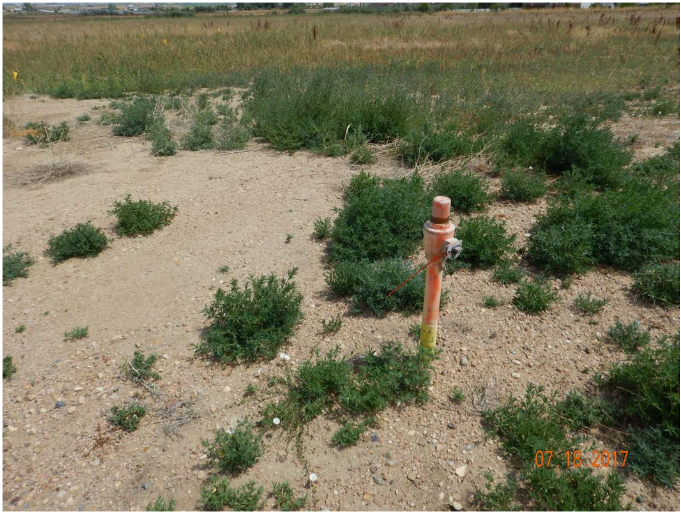
Photo 6 - Abandoned flowline riser, painted and tagged to comply with Flowline NTO.
