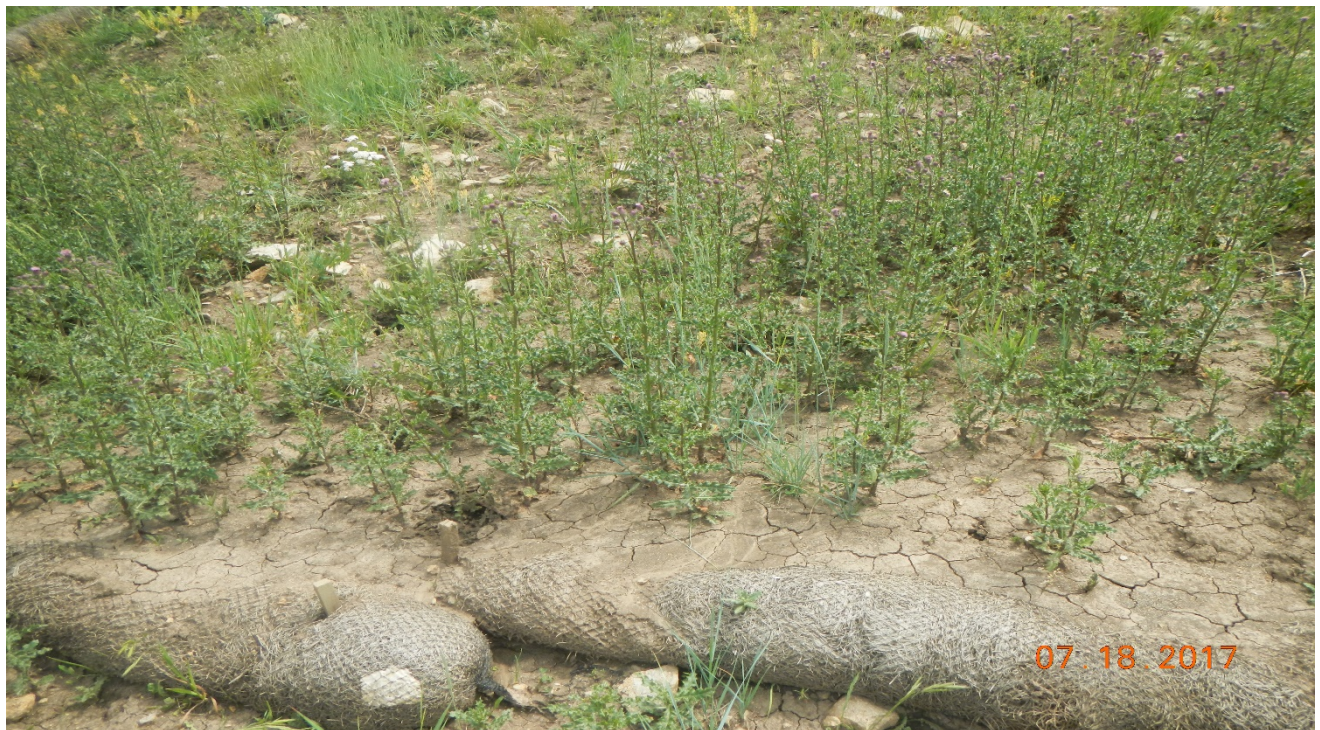
photo 4: The wattles along the slope have filled in with sediment and there are noxious weeds (Canada thistle along the south slope).
