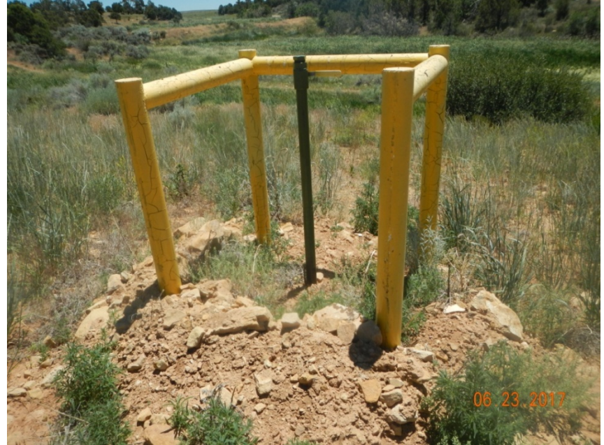
Photo 2: View of a second riser at 37.63208, -108.77241. This riser appears to be associated with the former well and is not locked or tagged out.
