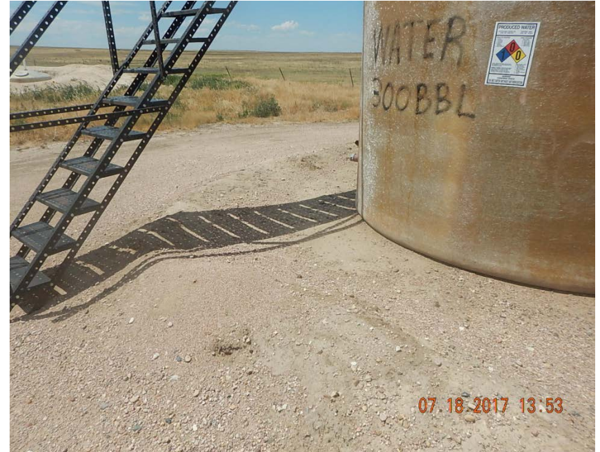
Photo 7: Inadequate berms at produced water tank
