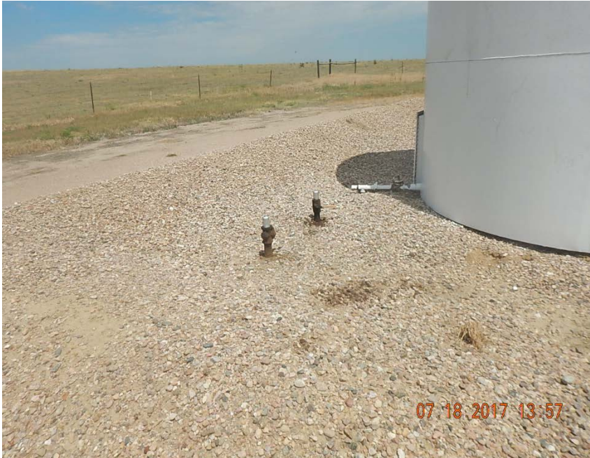
Photo 11: Disconnected risers at crude oil tanks
