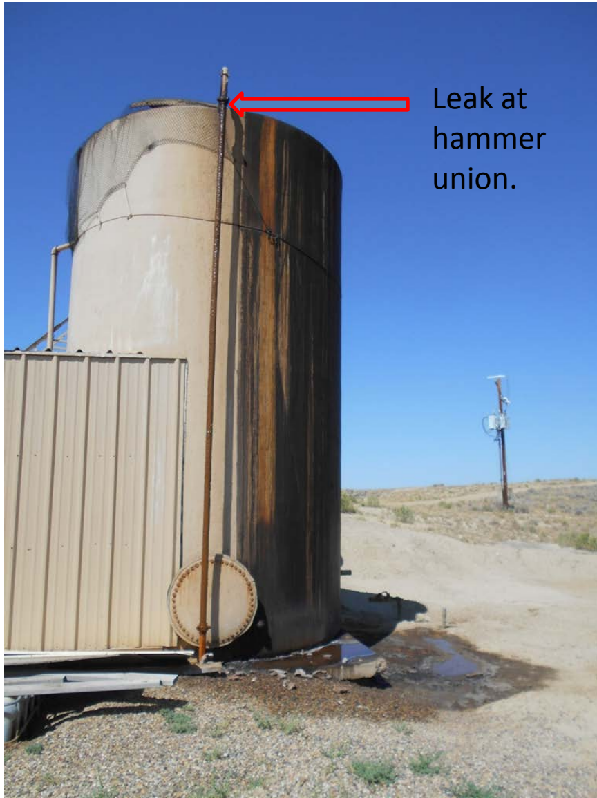
Tank Fill Line leak
