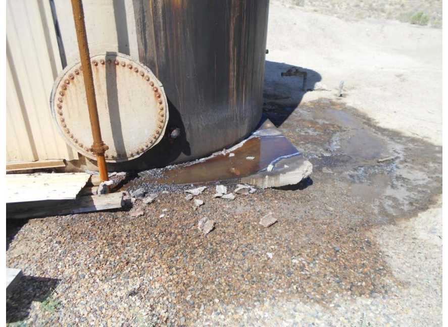
Tank Fill Line leak
