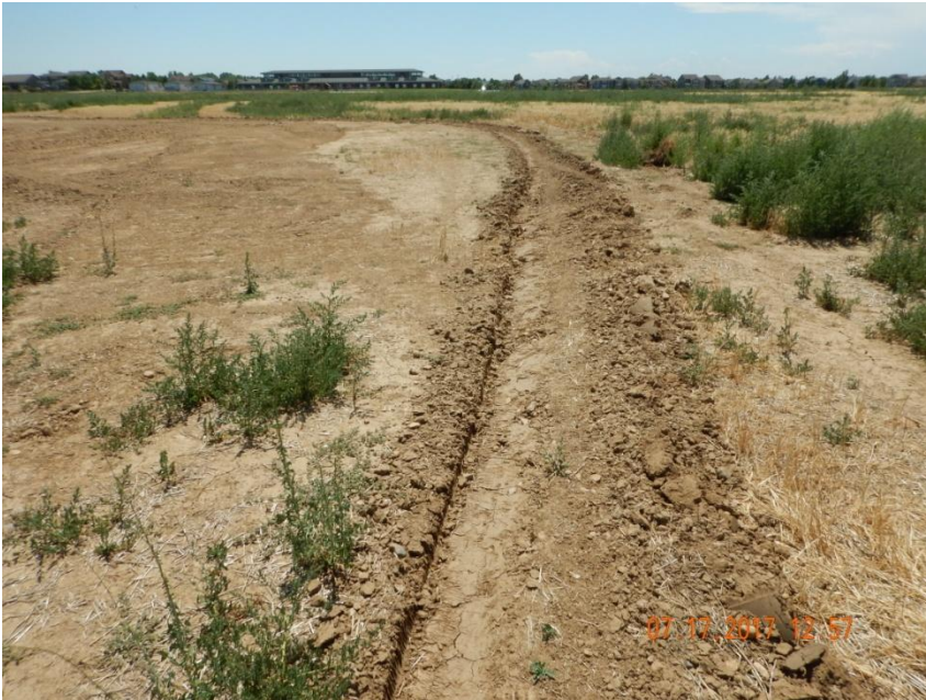
Photo 3. Photo taken from the western location, facing South. Surface roughening was performed around the location perimeter.
