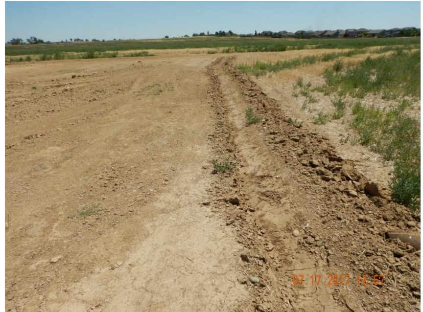
Photo 4. Photo taken from the southern location, facing East. Surface roughening was performed around the location perimeter.
