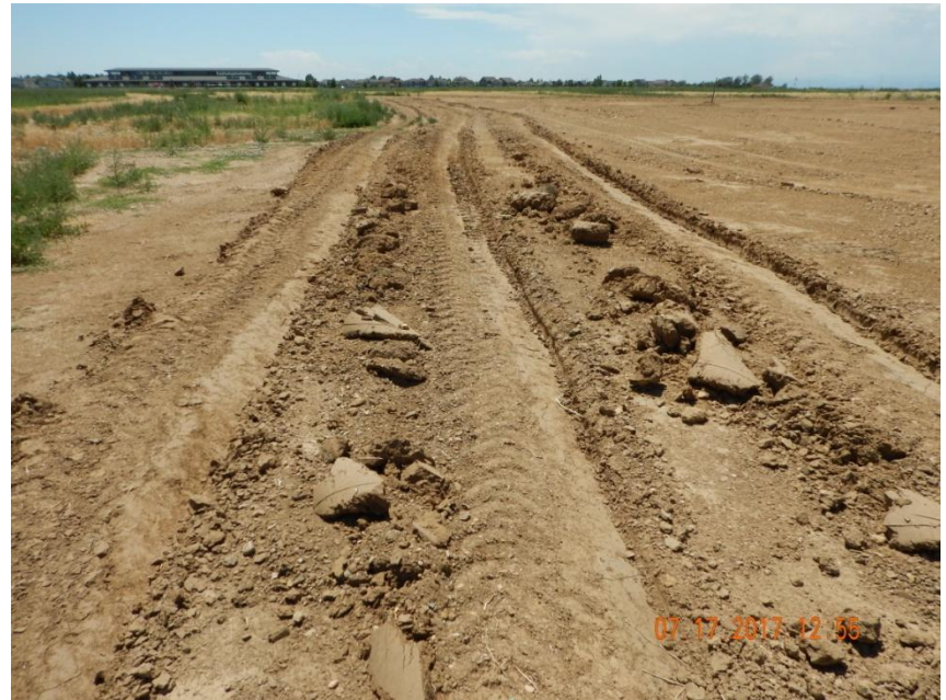
Photo 2. Photo taken from the northeast location, facing South. Surface roughening was performed around the location perimeter.
