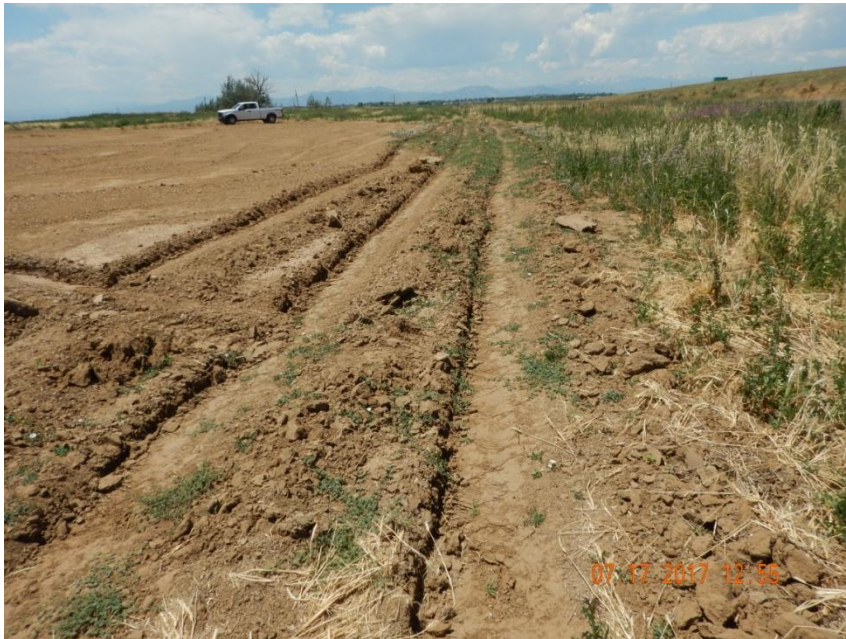
Photo 1. Photo taken from the northeast location, facing West. Surface roughening was performed around the location perimeter.
