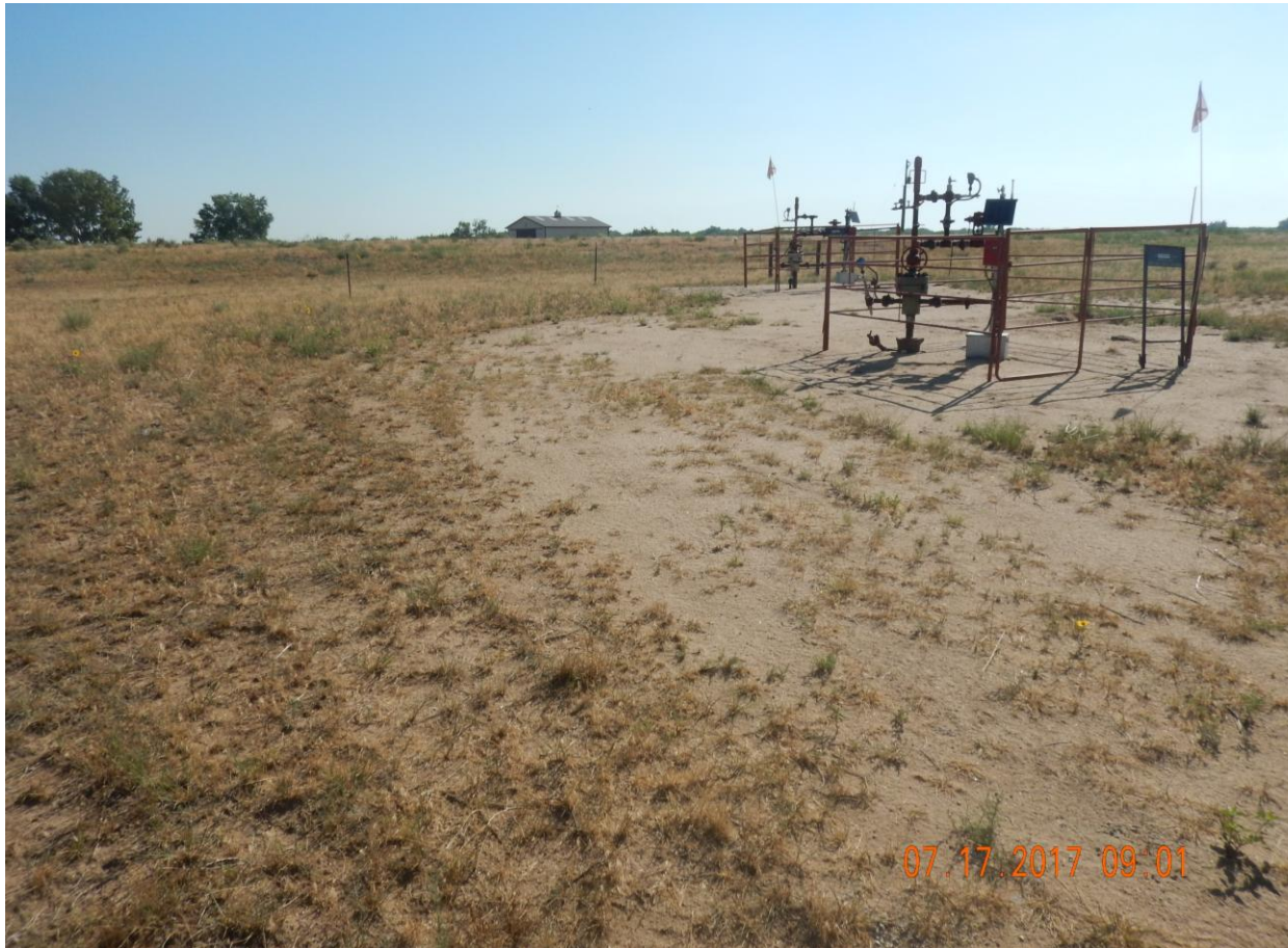
Photo 1: Multi well location. Well 123-18105 Pad, photo shows only two wells remain on location. PA'd well has been removed.
