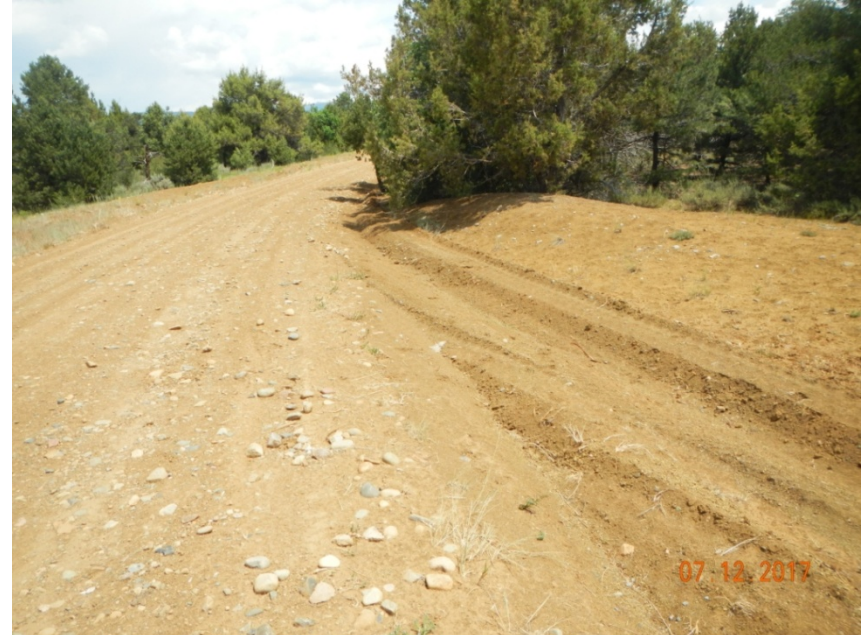
Photo 6: View of recently maintained roadside drainage on the access road. Soils are exposed and sediment controls are not in place.
