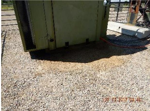
**Photo 7: Spill at OilLift unit.**
