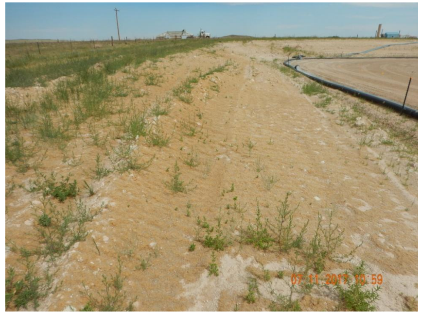
Photo 9. Photo taken from the western perimeter of the location, facing North. Cut slope appears to be stabilized with hydromulch but is only a temporary BMP.
