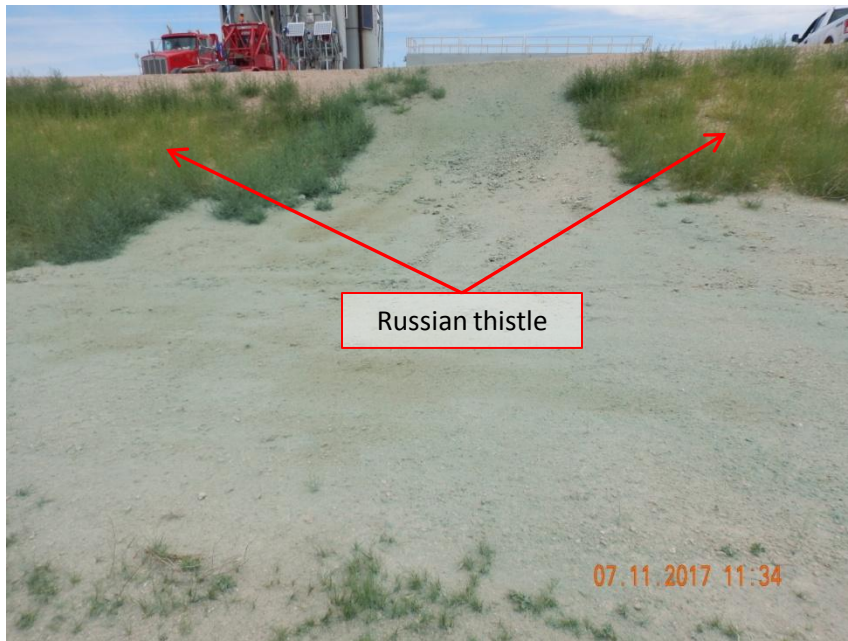
Photo 5. Photo taken from the southern perimeter of the location, facing North. Appears repairs have been conducted based off lack of vegetative growth, recent hydromulch application, and evidence of sediment discharge beyond the perimeter ditch and berm BMP.
