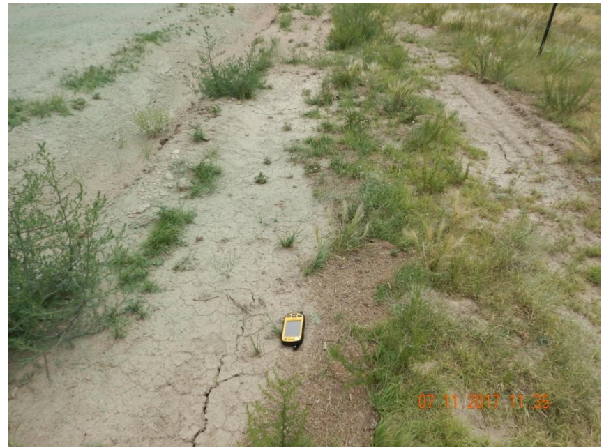
Photo 6. Photo taken from the previous photo location, facing East. Photo illustrates stormwater runoff appears to be washing sediment over the ditch and berm BMP off location. Refer to photo 7 for more detail.
