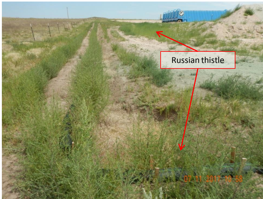
Photo 8. Photo taken from the southeast location, facing West. Sediment trap size was measured at ~6'x6'x2' (width x length x depth= 72ft 3 ) with filtrex at the overflow point of the trap.
