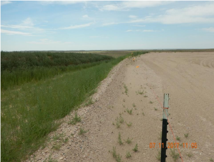
Photo 10. Photo taken from the eastern pad, facing South. A berm ~18" has been constructed along the west, east and south pad perimeter, but does not appear to be properly compacted.
