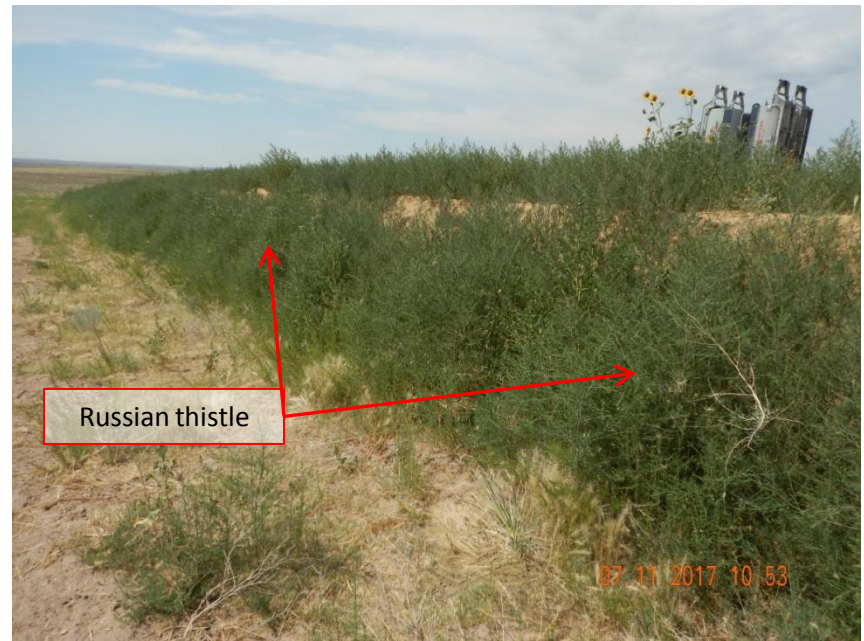
Photo 2. Photo taken from the eastern pad by the topsoil stockpile, facing South. Topsoil stockpiles were left with steep sides making it difficult to seed into for long-term stabilization and to prevent weed establishment.
