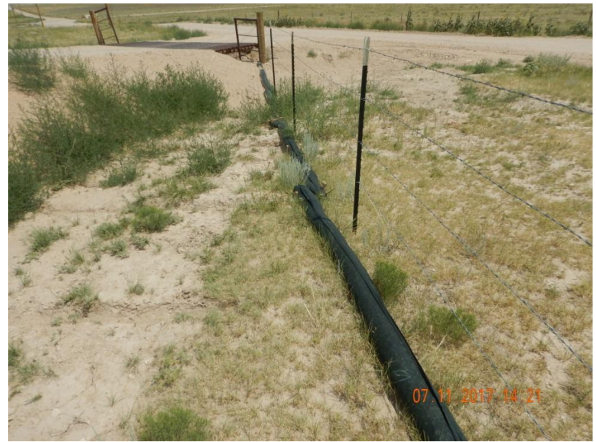
Photo 14. Photo taken from the east well pad, east entrance along the west side, facing East. Filtrexx wattle was installed beyond the outlet area to control runoff from the entrance of the access road which appears to be properly functioning.
