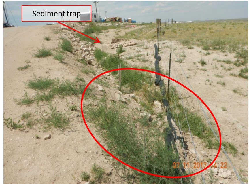
Photo 16. Photo taken from the east well pad, east entrance along the east side, facing Northwest. Appears stormwater runoff from the entrance access road is causing sediment discharge and the filtrex BMP does not appear to be a sufficient BMP.
