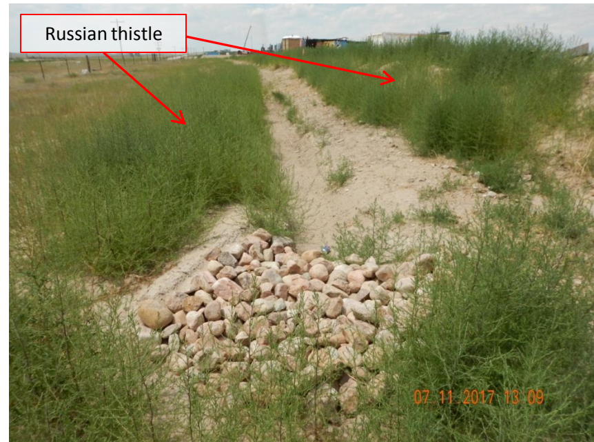
Photo 4. Photo taken from the west well pad, east entrance, facing West. Operator has installed a stabilized outlet at the end of the perimeter ditch but no sediment trap. Filtrexx wattle was installed beyond the outlet area to control runoff from the entrance of the access road but was not included because it was difficult to observe with the high density of Russian thistle. Refer to the next photo taken from the same area but on 4/3/2017.
