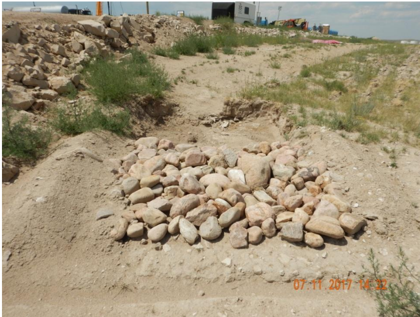
Photo 15. Photo taken from the east well pad, east entrance along the east side, facing Northwest. Sediment trap size was measured at ~6.5'x5'x1' (width x length x depth= 32.5ft 3 ) with a stabilized outlet. Fence line has been moved to facilitate maintenance for the sediment trap.
