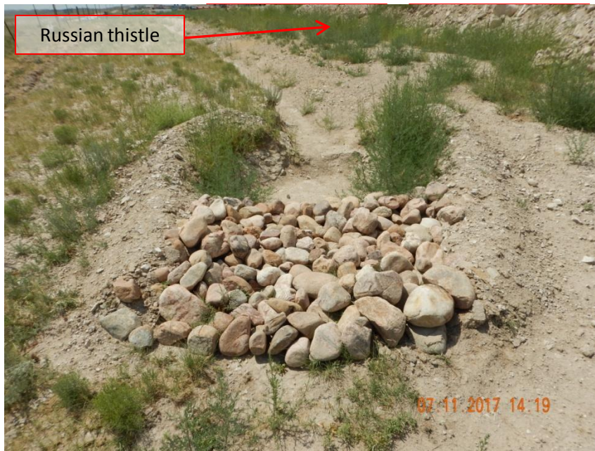
Photo 13. Photo taken from the east well pad, east entrance along the west side, facing West. Sediment trap size was measured at ~5'x4.5'x1.5' (width x length x depth= 33.75ft 3 ) with a stabilized outlet.
