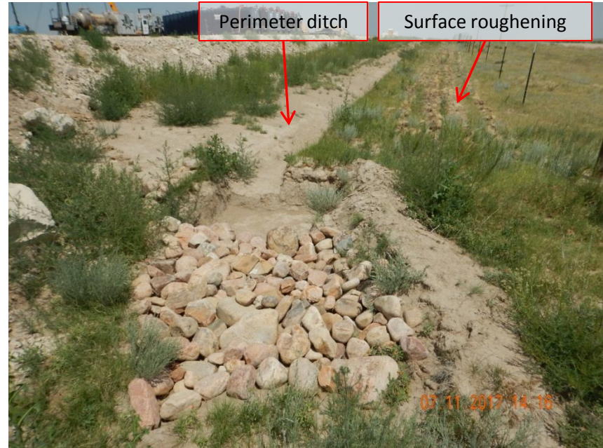
Photo 12. Photo taken from the southwest east well pad, facing East. Sediment trap size was measured at ~5'x4.5'x2' (width x length x depth= 45ft 3 ) with a stabilized outlet. Surface roughening outside of the perimeter ditch.
