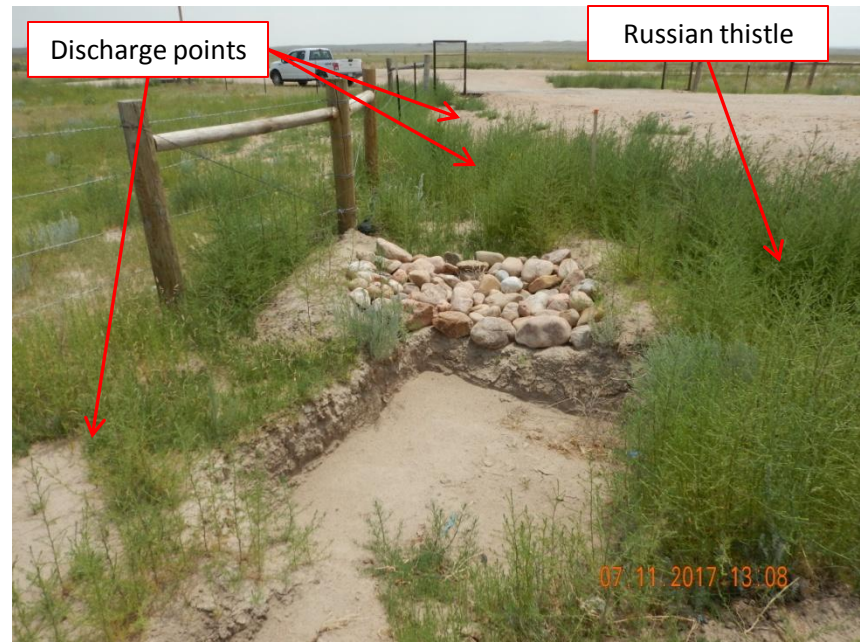
Photo 6. Photo taken from the west well pad, east entrance, facing South. Sediment trap does not appear to be sufficient as sediment is discharging from the eastern side. Sediment trap size was measured at ~5'x6'x1' (width x length x depth= 30ft 3 ) with a stabilized outlet. Sediment discharge is also occurring from the entrance of the access road, south of the sediment trap. Refer to photos 7 & 8.
