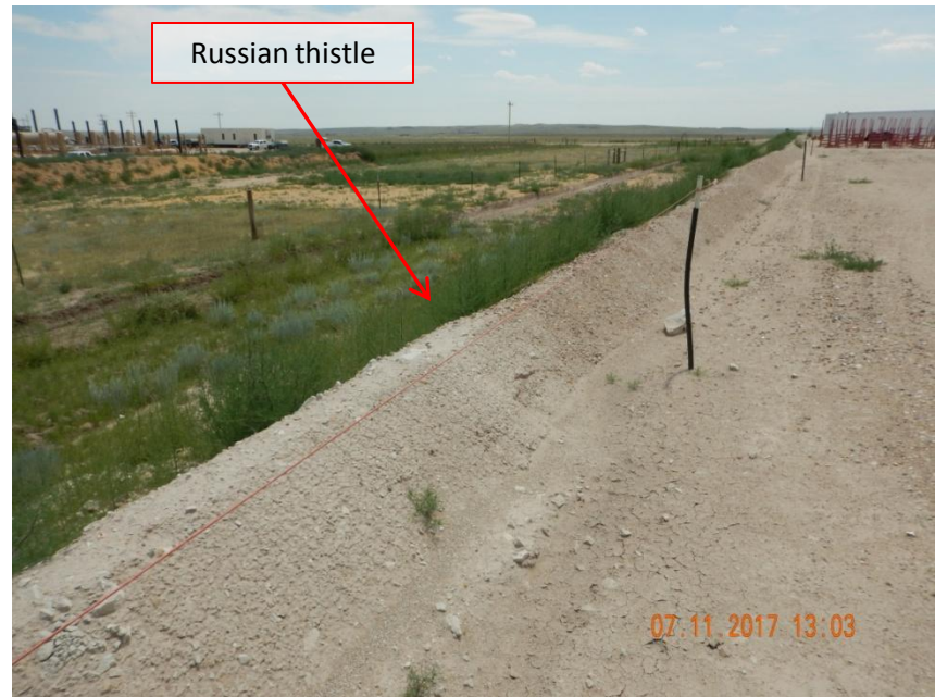
Photo 2. Photo taken from the eastern west well pad, facing Southeast. A berm ~18" has been constructed along the west, east and south pad perimeter, but does not appear to be properly compacted. Russian thistle growth was observed along the east-facing fill slope.
