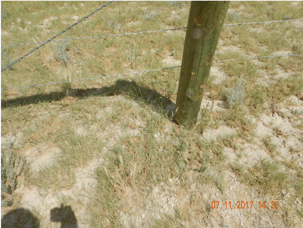
Photo 20. Close up photo taken just beyond the sediment trap, illustrating stormwater runoff appears to be washing hydromulch material off location.
