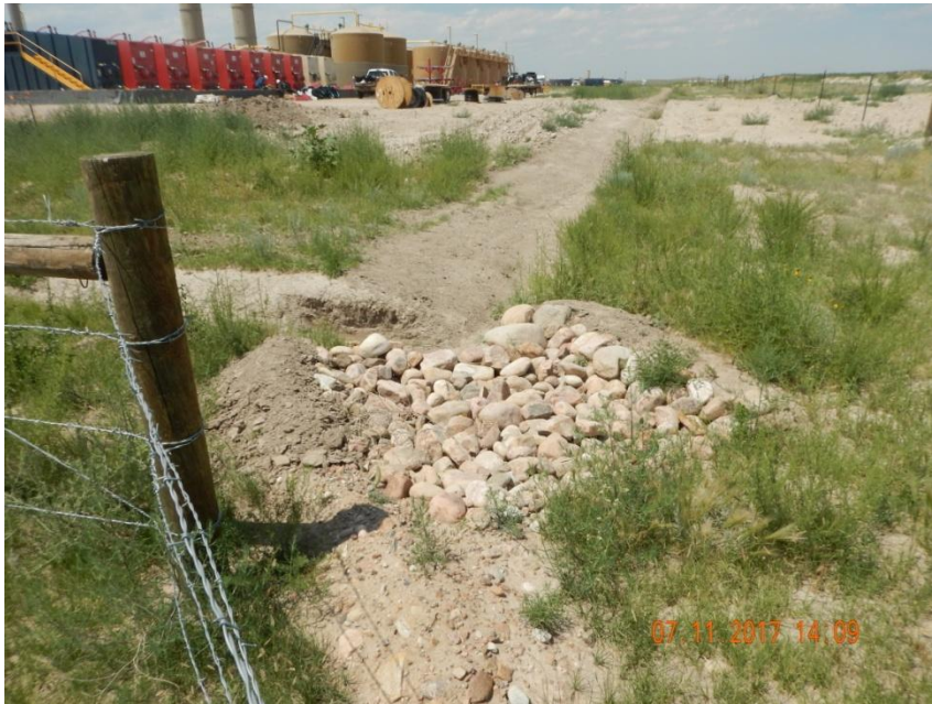
Photo 11. Photo taken from the southeast production facility pad, facing North. Sediment trap size was measured at ~5.5'x4'x1.5' (width x length x depth= 33ft 3 ) with a stabilized outlet.
