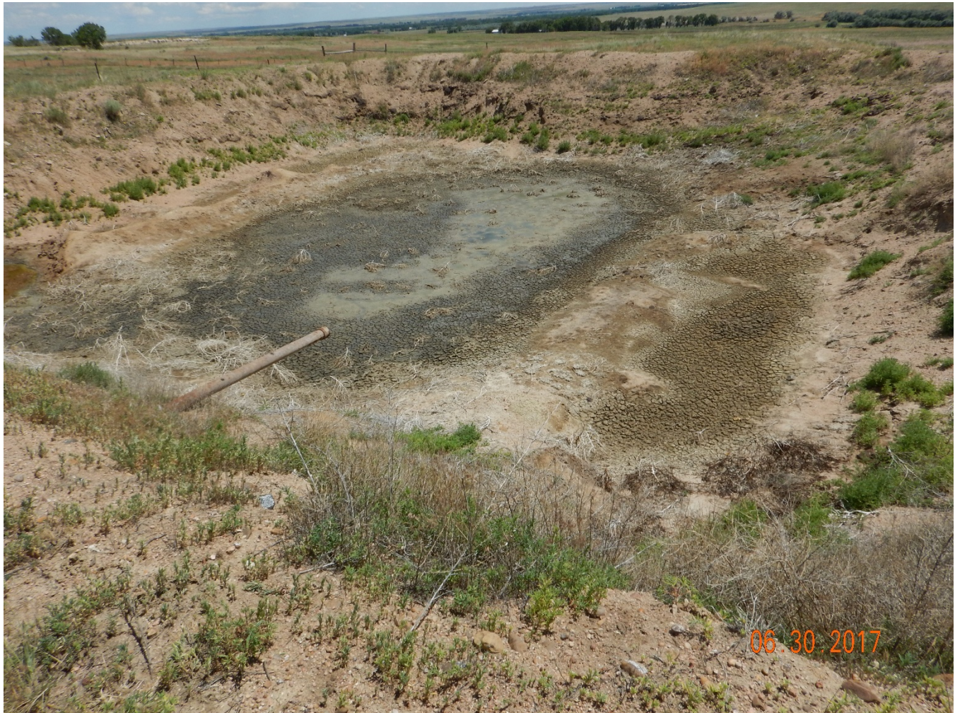
Figure 8 - Produced water pit remains on location. Operator indicated that both pits would be remediated by 6/15/2017.
