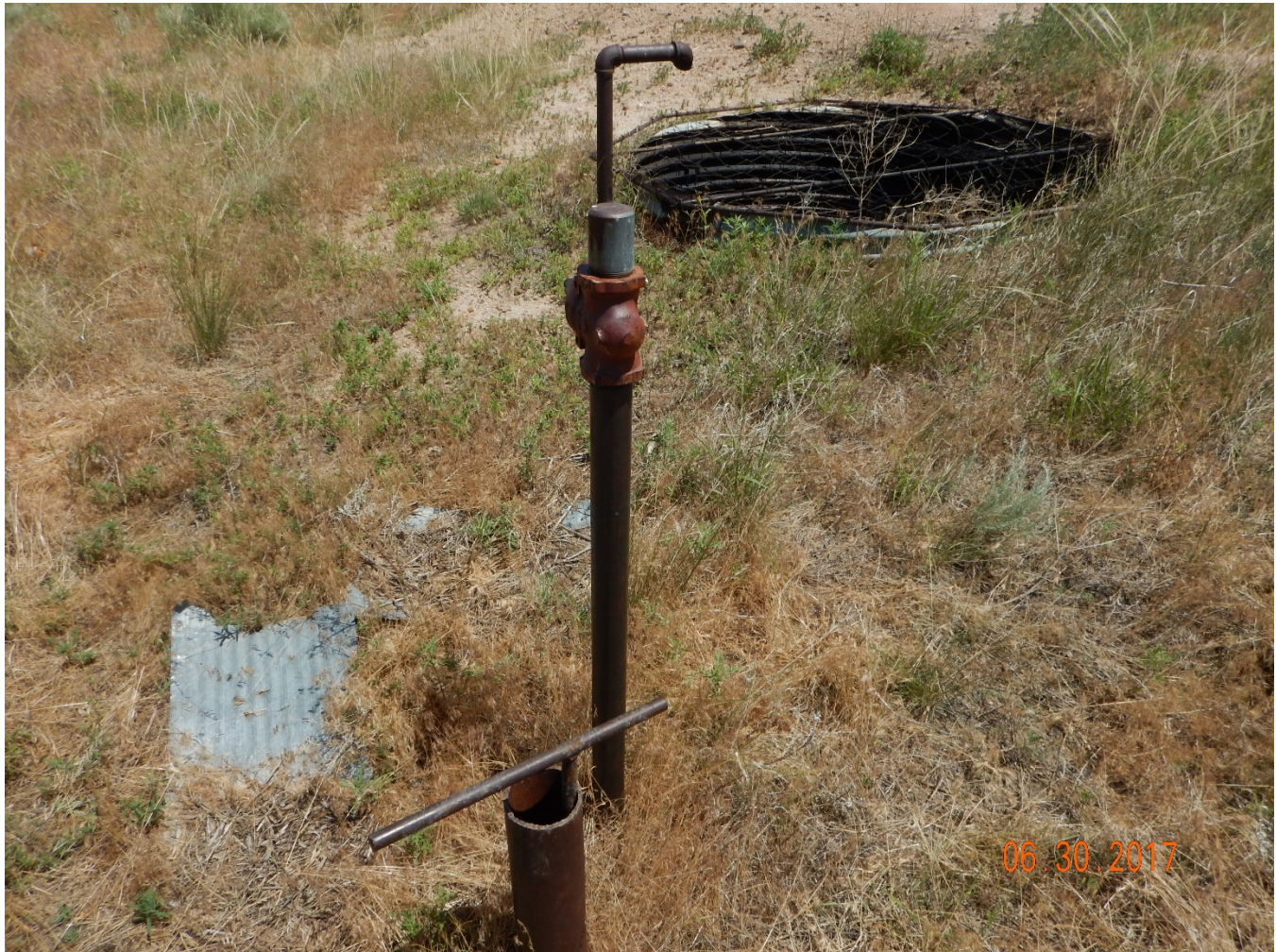
Figure 7 - Abandoned flowline risers N and NW of tinhorn.
