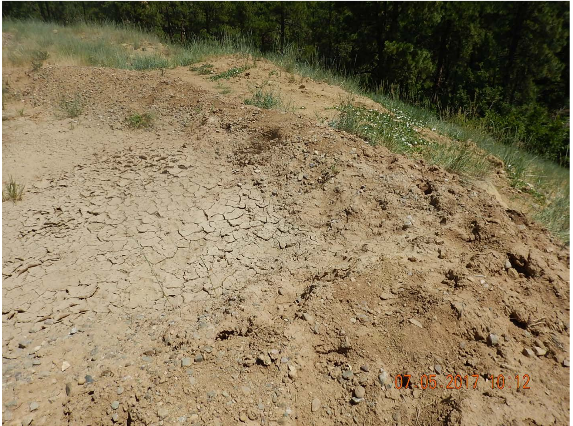
Down slope side of secondary containment berm. Berm was damaged during spill response.
