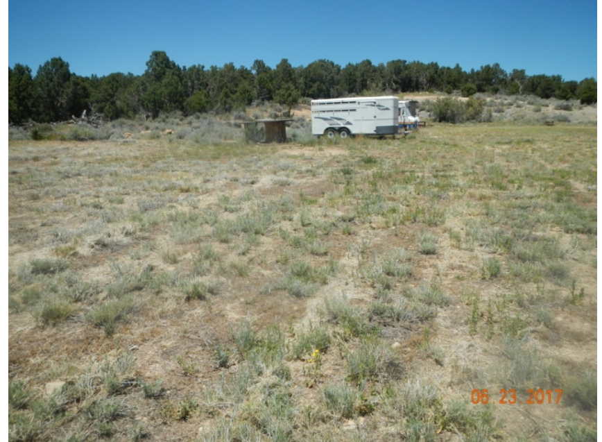
Photo 4: View of the western portion of the project area from the southwestern corner facing northward. Well pad is not recontoured. Vegetation is established and mowed. What appears to be surface owner equipment is stored in this portion of the well pad area.
