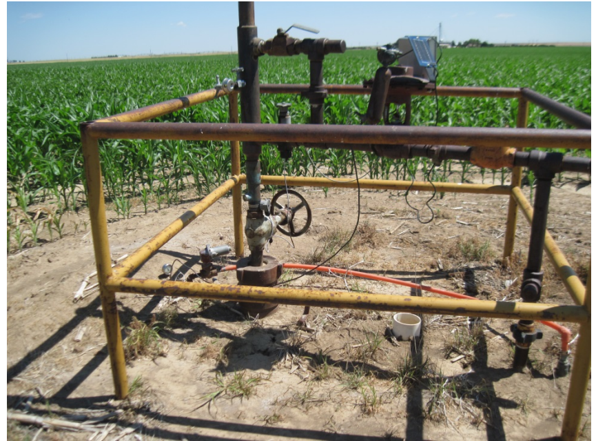
1" RISER AND PLASTIC REMOVED AND PLUGGED AT WELLHEAD
