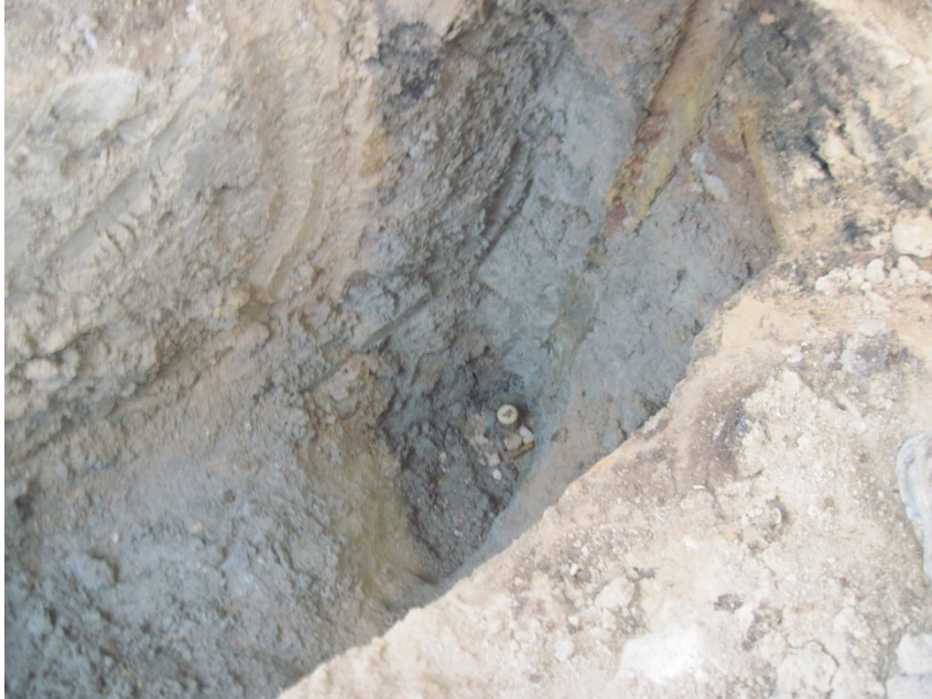
RISER PLUGGED OLD WATER LINE AT CRYSTAL-HUBBS #1 BATTERY
