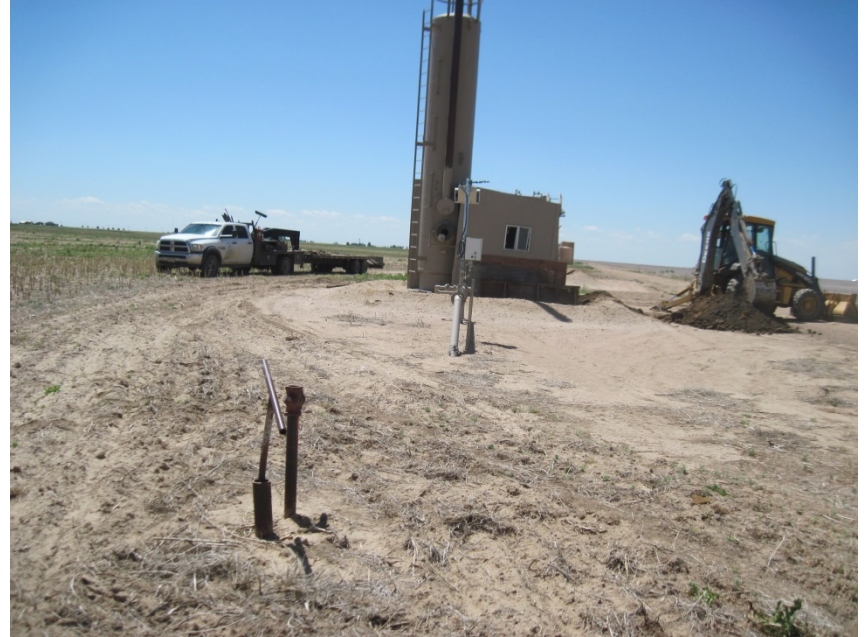
MARKED RISER ARE GOING TO BE REMOVED AND VALVE UNDERGROUND
