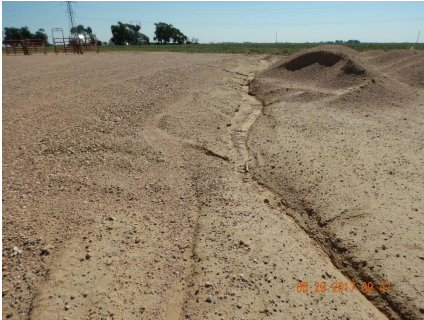
Photo 3. Photo taken from the southern location, facing East. Gully erosion is occurring adjacent to the location from stormwater and/or irrigation water run-on onto location.
