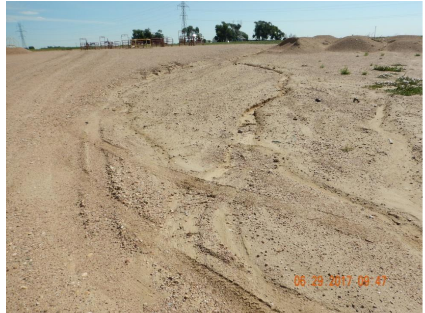
Photo 4. Photo taken from the area that would likely be the inlet of the culvert, facing East. Appears sediment has accumulated overtime blocking the inlet of a culvert-see following photo.
