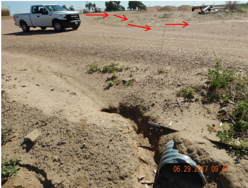
Photo 5. Photo taken from the outlet of the culvert along a portion of the access road, facing Northeast. Did not observe the inlet of the culvert due to sediment build up overtime. Red arrows indicate the likely direction of current water flow.
