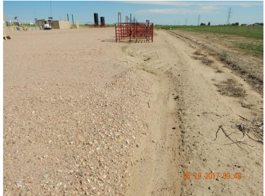
Photo 2. Photo taken from the eastern location, facing North. Gully erosion evident from stormwater and/or irrigation water run-on onto location.
