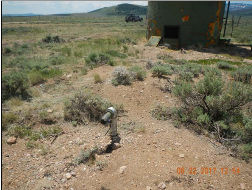
Photo 3. Steel riser not in use, not locked out tagged out.
