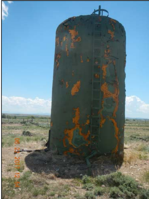
Photo 1. Insulated tank, no berm or labels.
