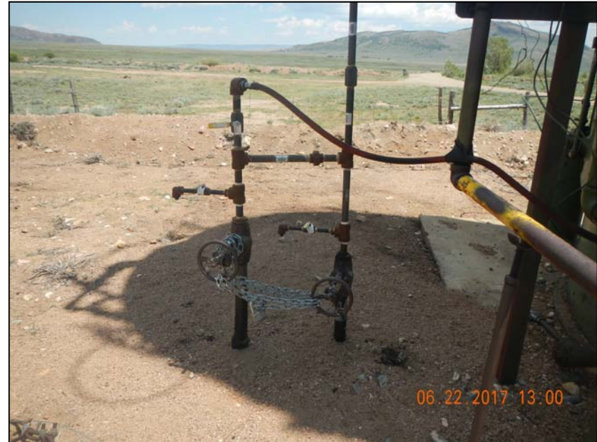
Photo 8. Steel risers not in use at separator not locked out tagged out.
