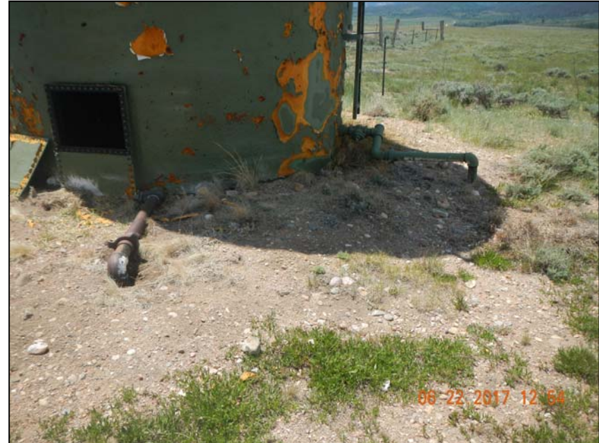
Photo 2. Risers at tank not in use, not locked out tagged out.
