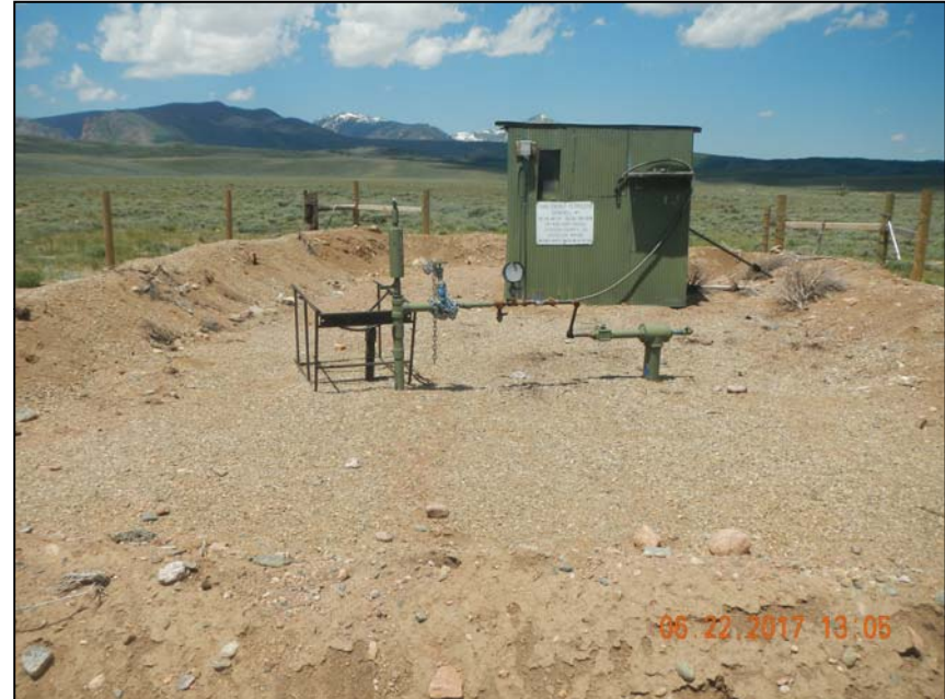
Photo 10. Steel risers not in use at wellhead not locked out tagged out.
