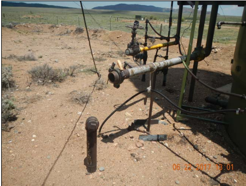
Photo 7. Steel riser not in use, not locked out tagged out in southern pit.
