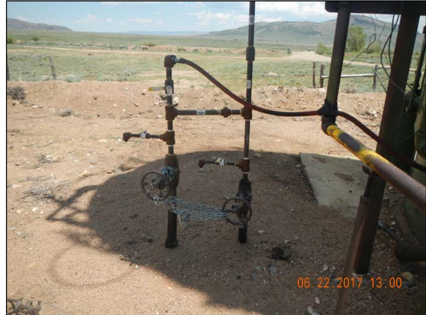
Photo 6. Steel risers at separators locked out tagged out.
