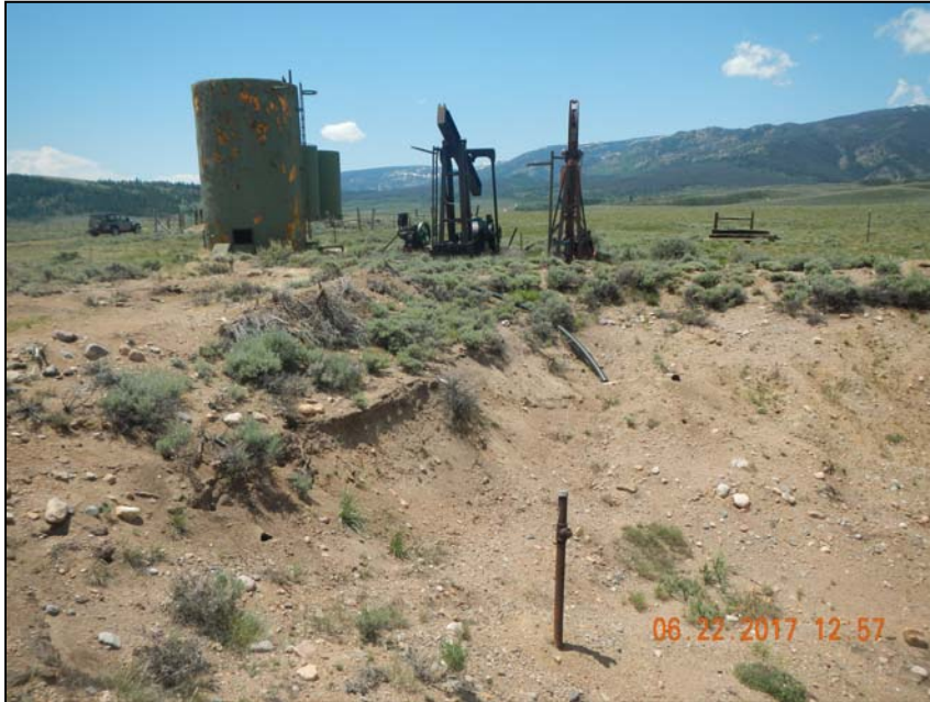
Photo 5. Steel riser not in use, not locked out tagged out in southern pit.
