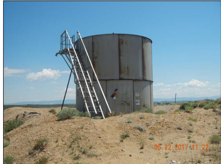
Photo 6. Tank label missing capacity.
