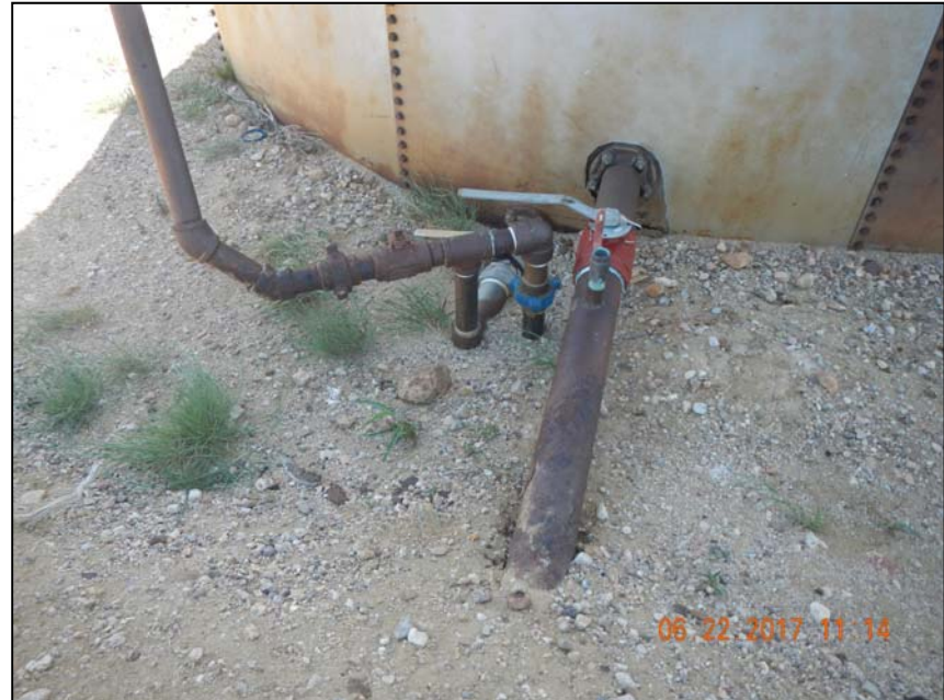
Photo 2. In Use riser at tank.
