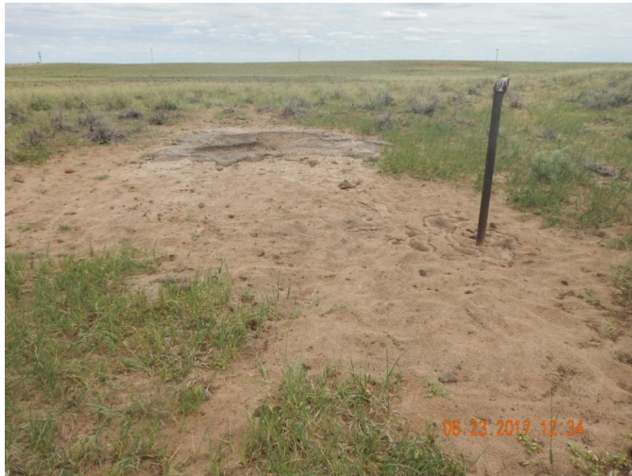
Photo 3: Photo taken from the north east end of the location, facing east. Photo shows pipe riser on location. Photo also shows a black, hard material staining the soil throughout the well location, pits and access road.
