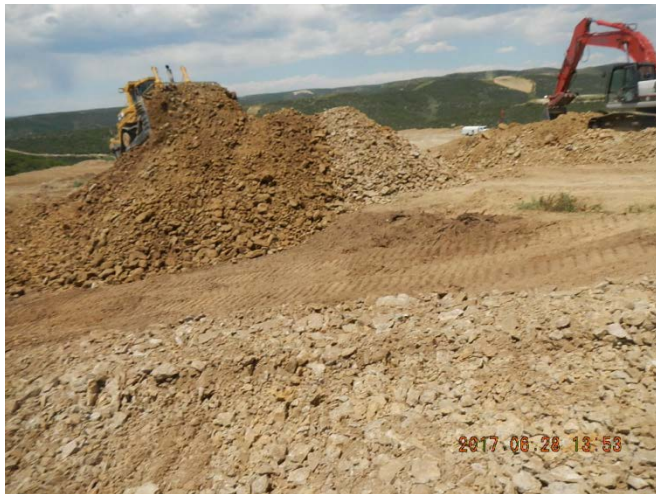
Overburden material being pushed with dozer.
