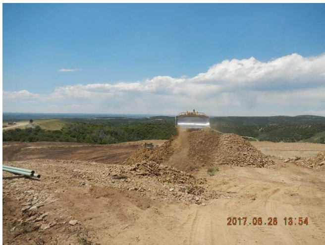
Overburden material being pushed with dozer.
