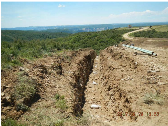
Trench, sandbags, pipe, fractured rock.
