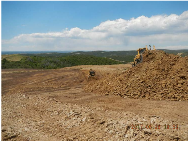
Overburden material being pushed with dozers.
