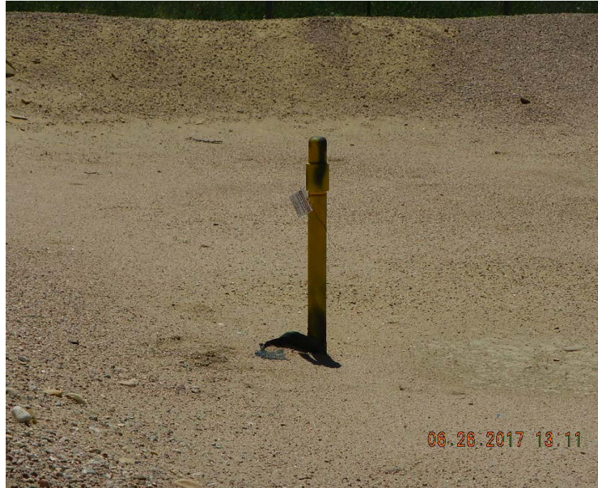
Unused marked and tagged out riser
