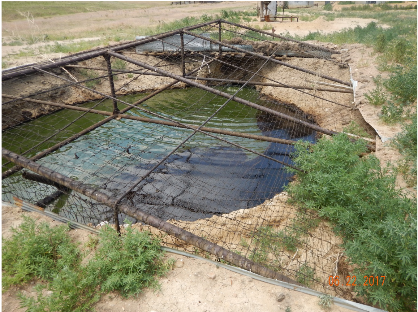
Figure 13 - Skim pit (COGCC Facility ID #104647). Wildlife mesh was in good shape on inspection date. Note: oil on pit, uncontrolled weeds in/out of berm, erosion of pit berm.
