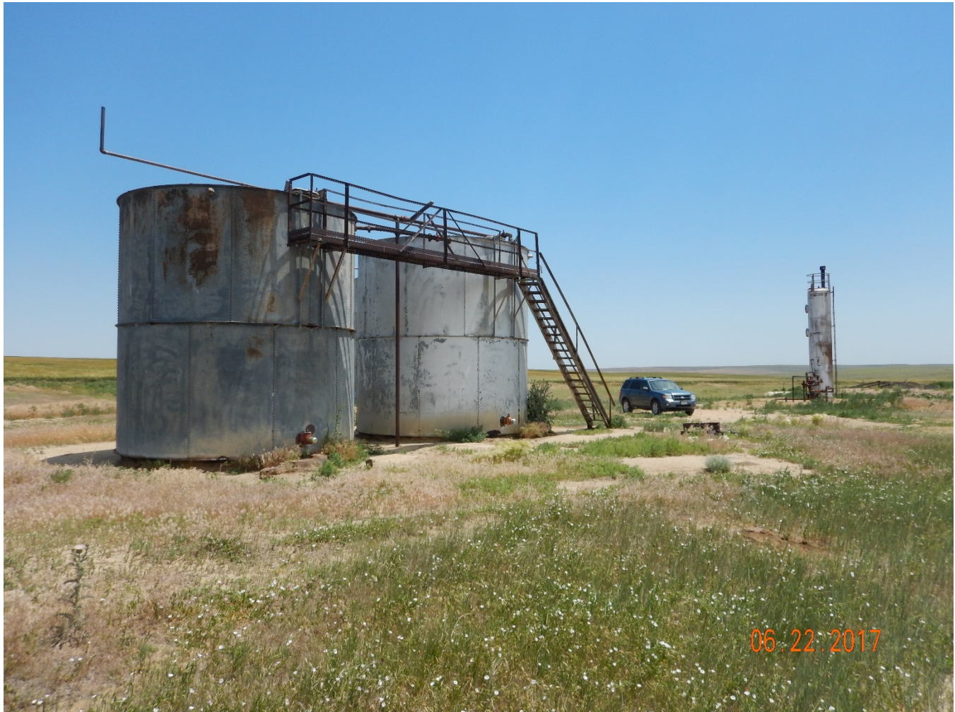
Figure 8 - Unidentified steel panel ASTs at NW corner of location lack volume and NFPA labels. Note complete absence of secondary containment.
