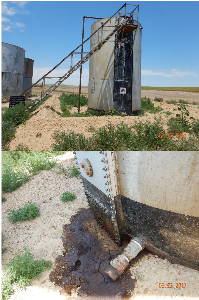
Figure 7 - Bermed, crude-oil AST (top) and close-up on exposed valve with oil-stained soil on NW side of tank. Note: uncontrolled weeds growing into berm.
