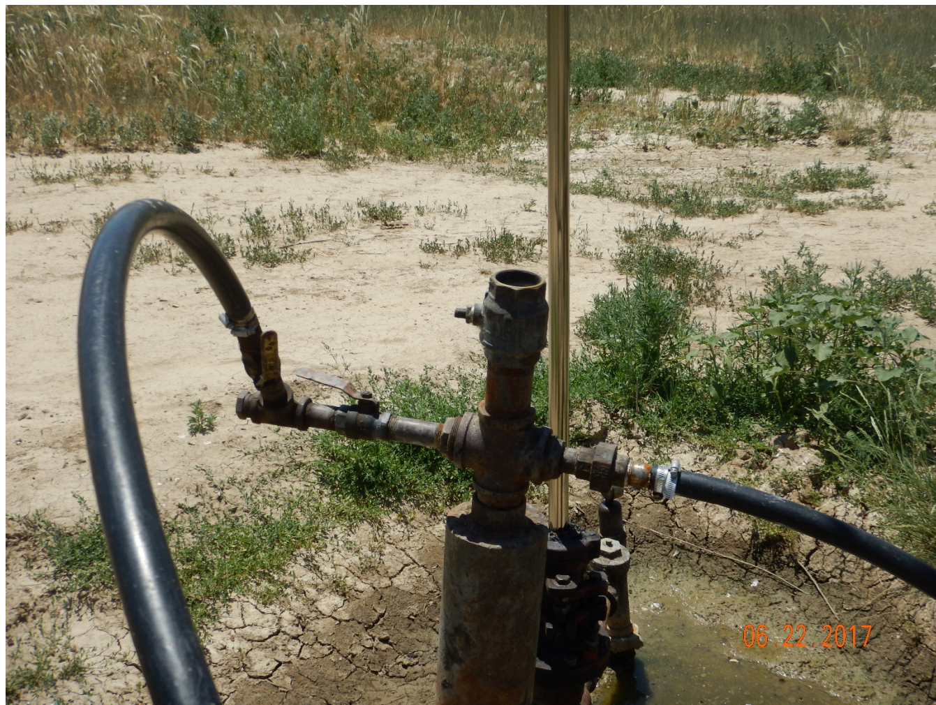
Figure 3 - Wellhead equipment is open to atmosphere (no bullplug installed).
