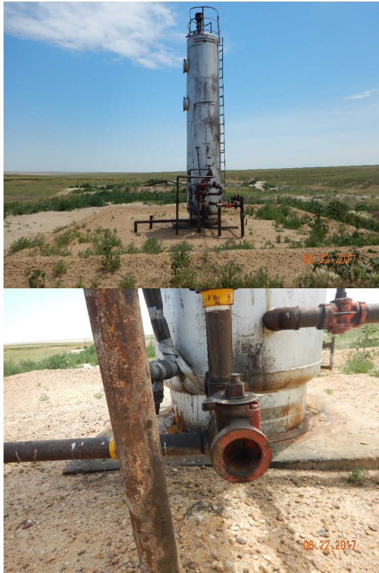
Figure 11 - Vertical heater treater with earthen berm (top) and close-up on exposed valve located on north side of treater (bottom). Note: uncontrolled weeds.
