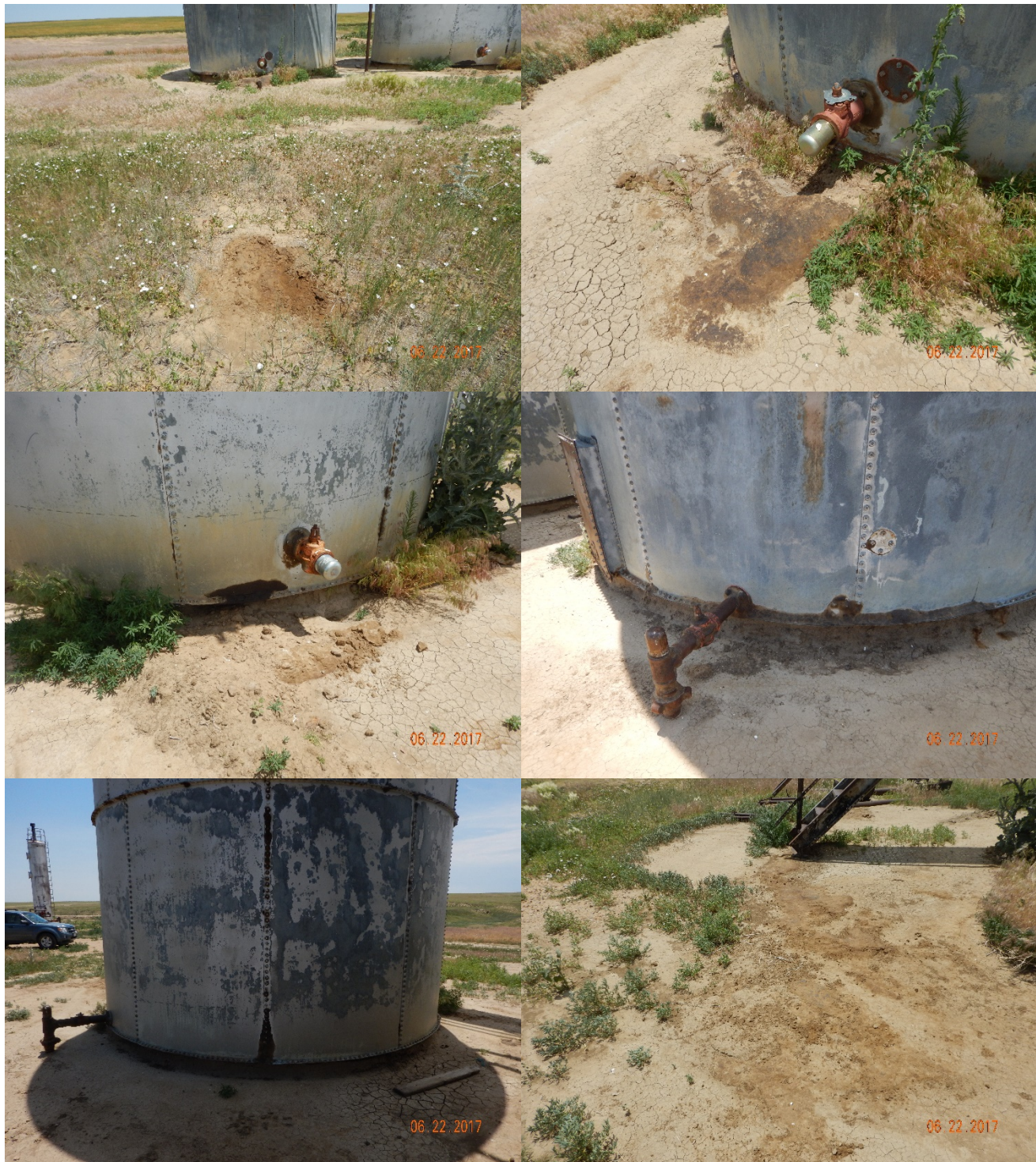
Figure 9 - Assorted shots of localized, oil-stained soil associated with unidentified tanks at former loadout west of tanks (top left), beneath valves on either side of tanks (top right, middle left & right), weeping from bolts (bottom left) and east of stairs (bottom right).
