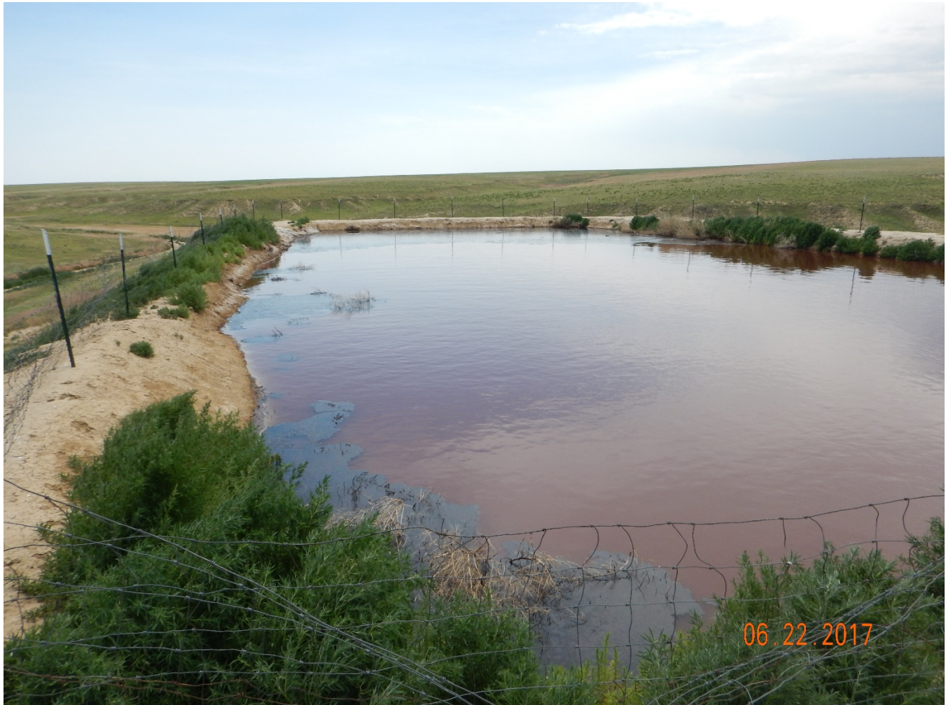
Figure 14 - Produced water pit (COGCC Facility ID #114378). Note: uncontrolled weeds and erosion of pit berm. Oil is present around perimeter of pit.
