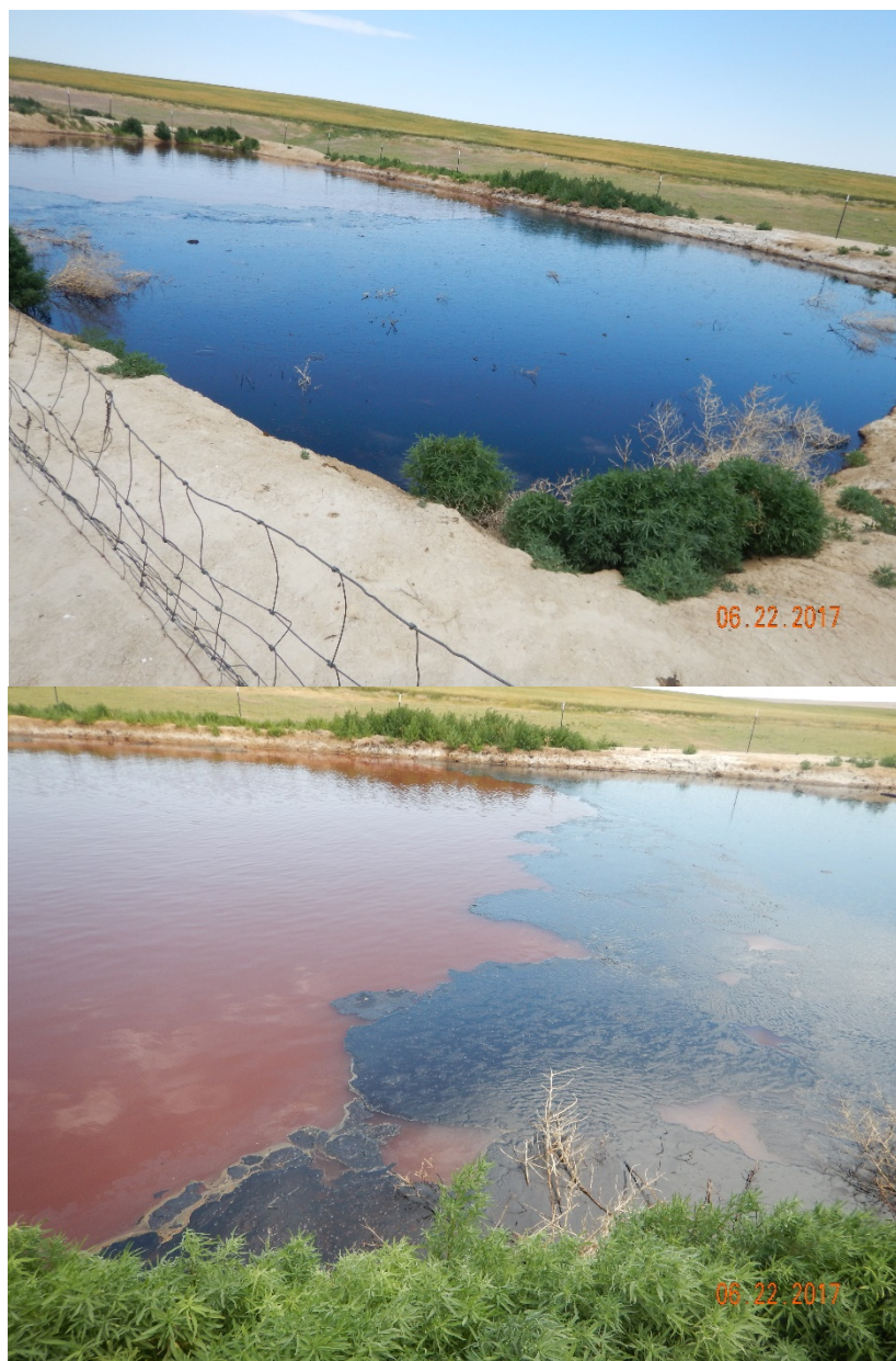
Figure 15 - Oil covers south end of produced water pit (top) and close-up of water/oil contact (bottom).
