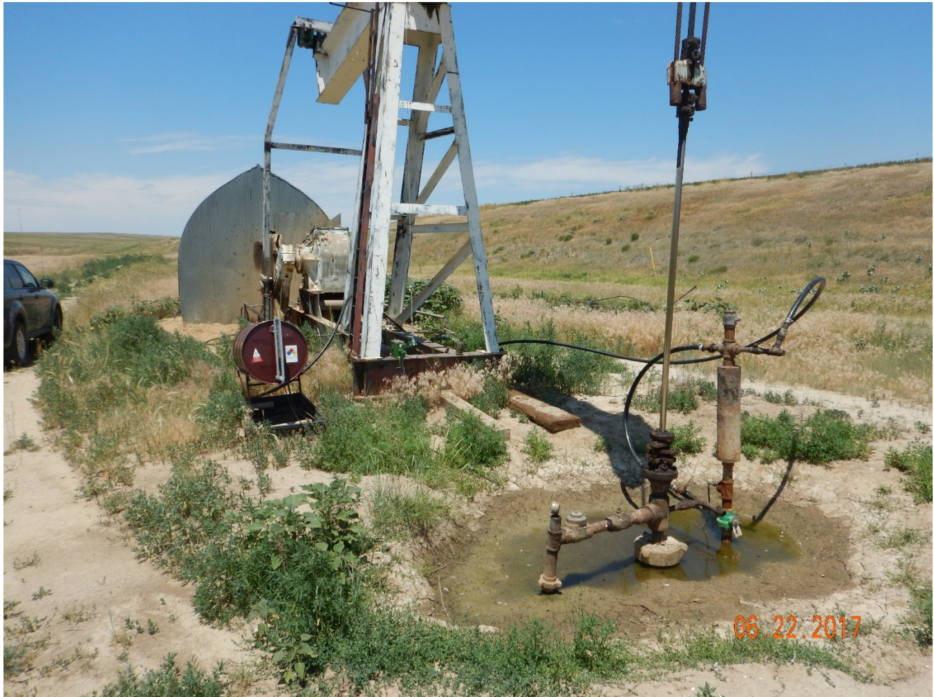
Figure 2 - Price-Degenhart 1 Wellhead. Note: puddle/depression around wellhead, uncontrolled weeds, and chemical storage tank.
