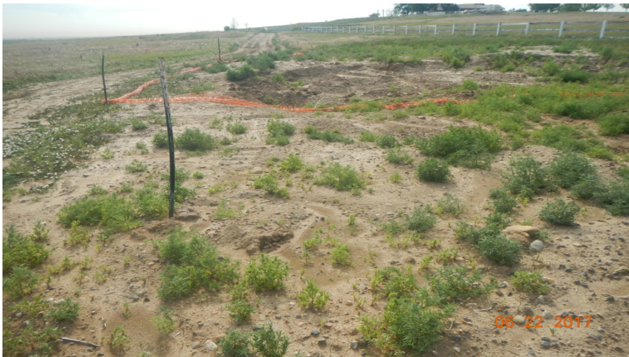
photo 6: Facing east at tank battery site. There is an area of subsidence and the orange safety fence is not maintained.
