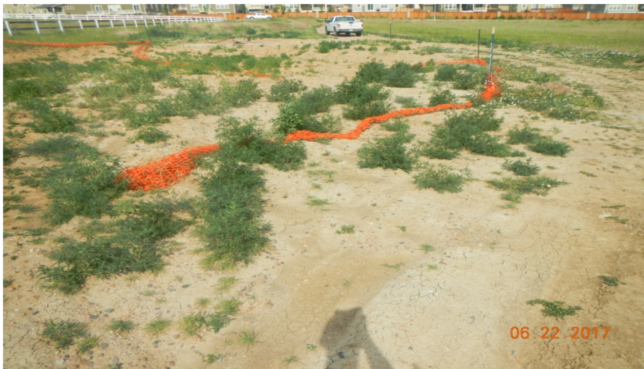
photo 7: Facing west at the tank battery site. There is an area of subsidence and the orange safety fence is not maintained.
