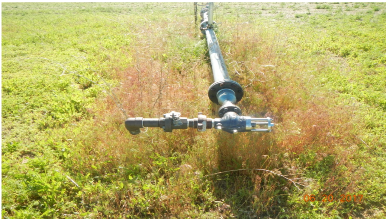
photo 8: One end of the pipe riser has been disconnected, capped and locked out.
