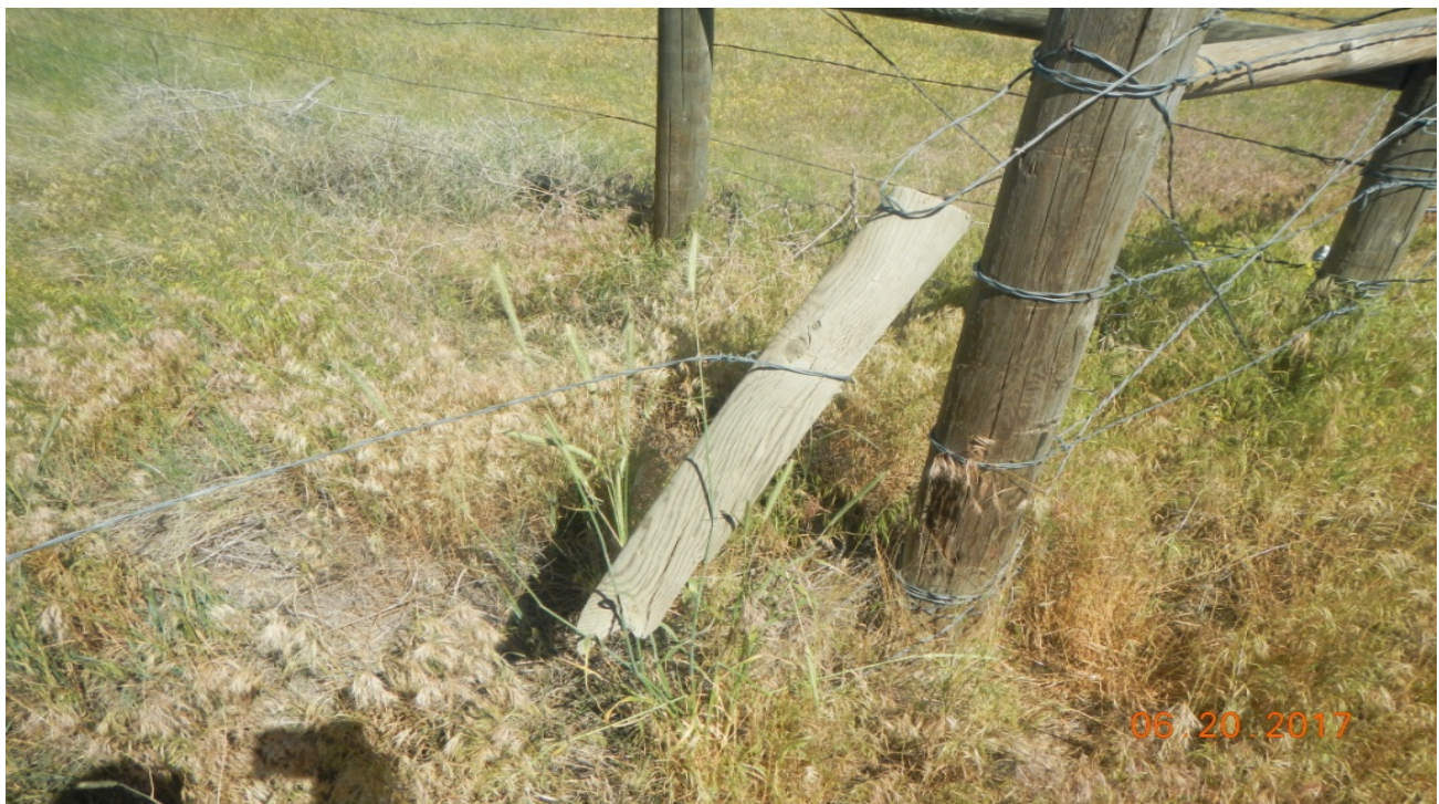
photo 2: The gate at the fenced site is broken and need to be repaired.
