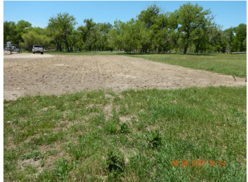
Photo 2. Photo taken of the northern location, facing West. Area inside the guy line anchors were sprayed to control weeds, then seeded and hydromulched.
