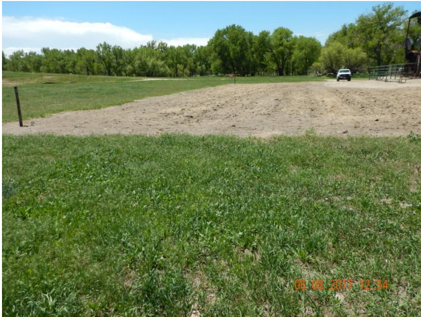
Photo 1. Photo taken of the southern location, facing West. Area inside the guy line anchors were sprayed to control weeds, then seeded and hydromulched.
