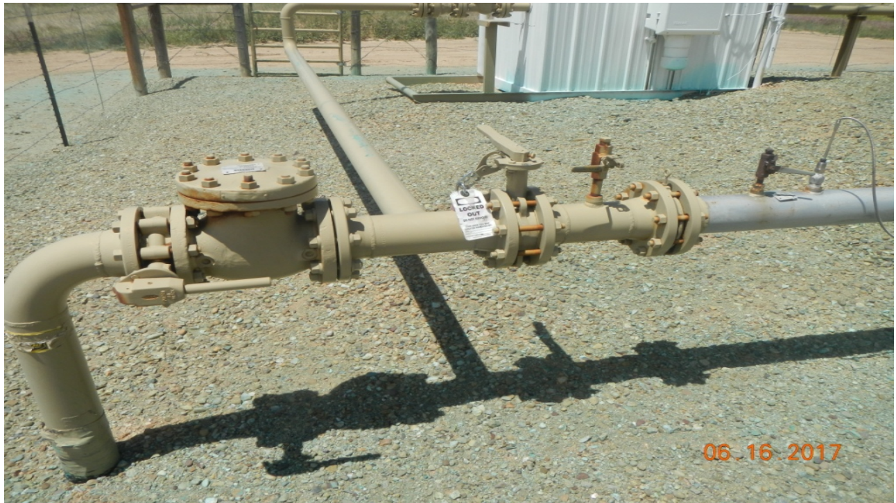
photo 3: This valve on the pipe line lever has lock out/tag out.
