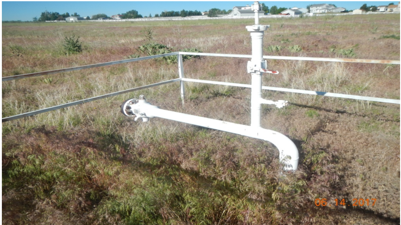
photo 3: There is no lock out/ tag out applied to this pipe riser.
