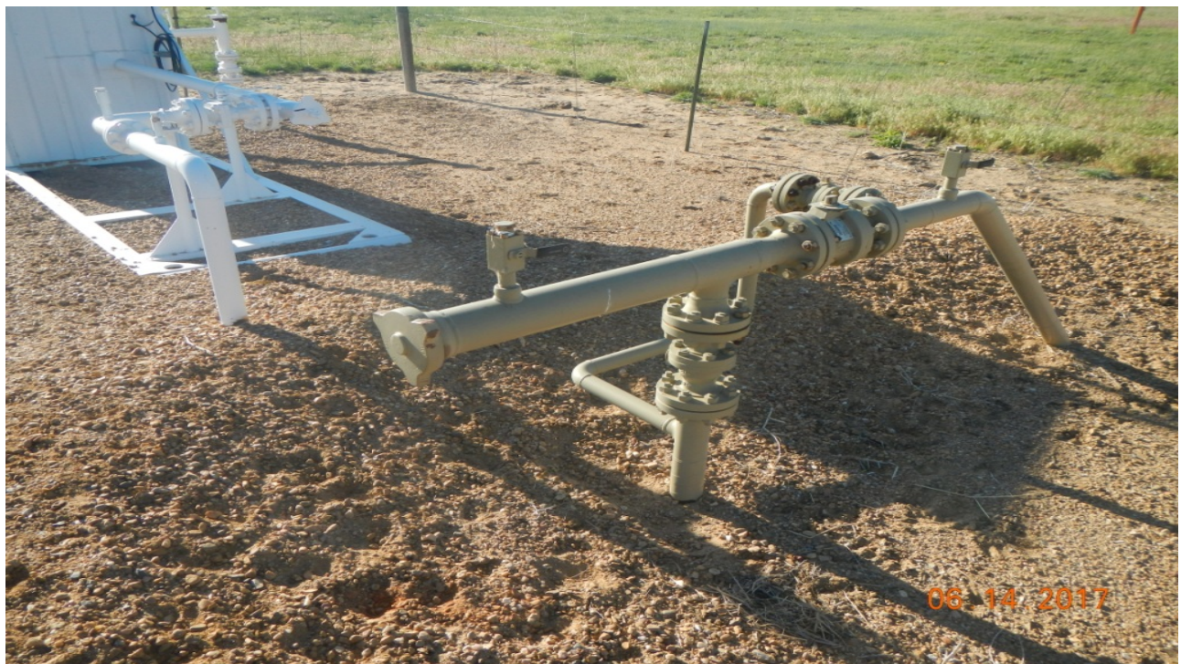
photo 6: There is no lock out/tag out that has been applied to the pipe infrastructure.
